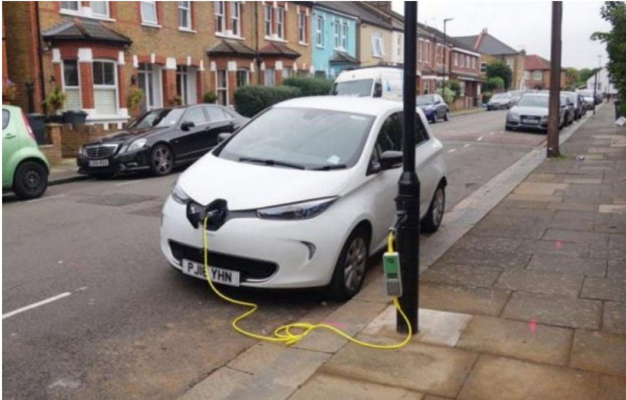
Figure 4: Example of On-Street Lamppost Charger
