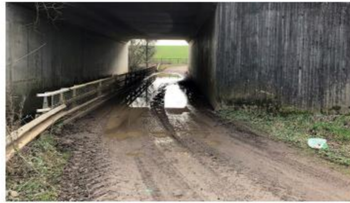
Unsurfaced underbridge of A43 PROW link to Whitfield
