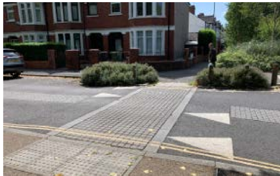
Build outs can serve a number of uses including formalising on-street parking and creating traffic calming effect by narrowing the carriageway. They can also provide opportunities for crossing points on raised tables.
