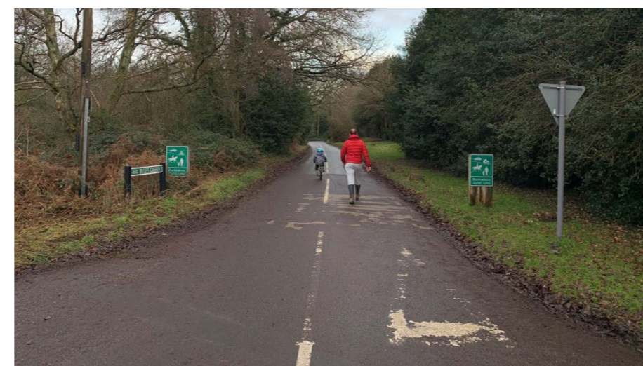
Quiet Lane designations combined with rural traffic calming can encourage slower speeds and courteous behaviour on quiet rural lanes where pedestrians, cyclists and horse riders need to share the space with vehicles
