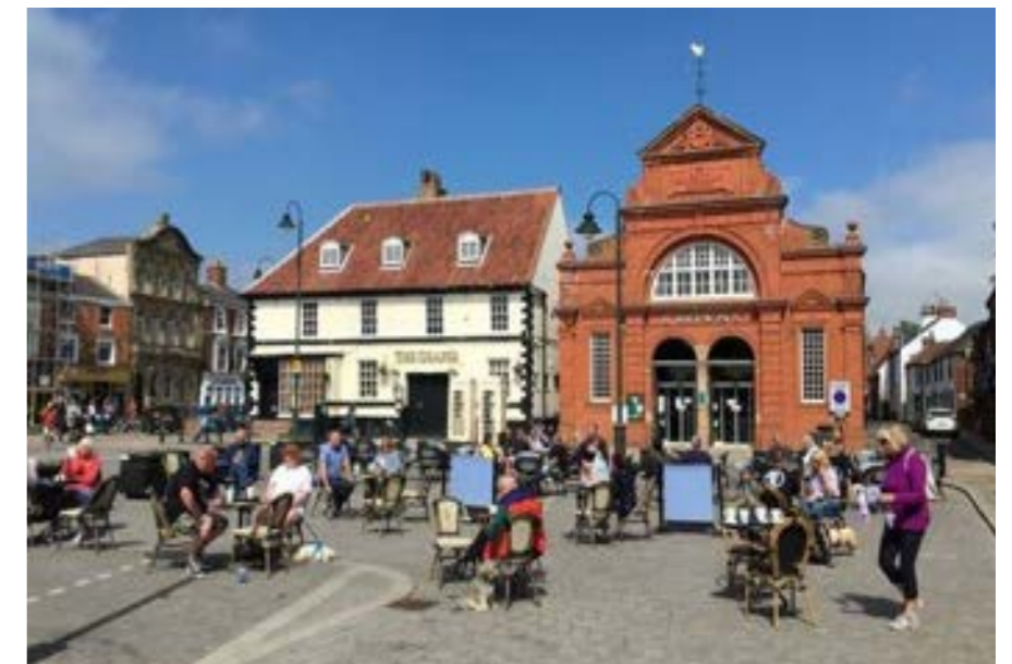
Areas can be designed to be used flexibly e.g. car parking, markets, events (Beverley)
