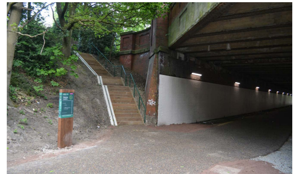
Providing lighting and a suitable width through underpasses is important to improve feelings of personal security (Tyldesley Loopline, Salford)
