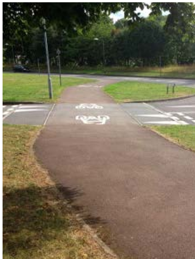
Tightening junctions and providing pedestrian and cycle priority – either by design or marked priority – provides a higher level of service for pedestrians and cyclists travelling along a main road
