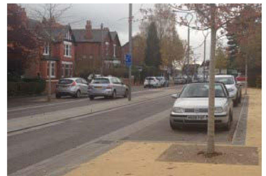
Central reservation and inset parking bays visually narrow the carriageway and encourage slower speeds (Poynton)
