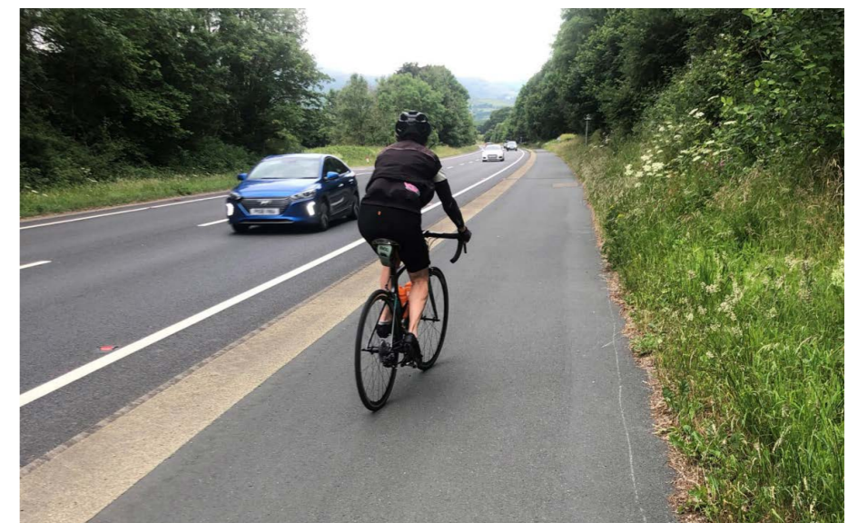
Shared use foot/cycleways can provide a good level of service for both pedestrians and cyclists on rural roads as well as some suburban roads which have few or no active frontages or driveways. A buffer should be provided between the road and the shared use facility on roads with speeds over 30mph.
