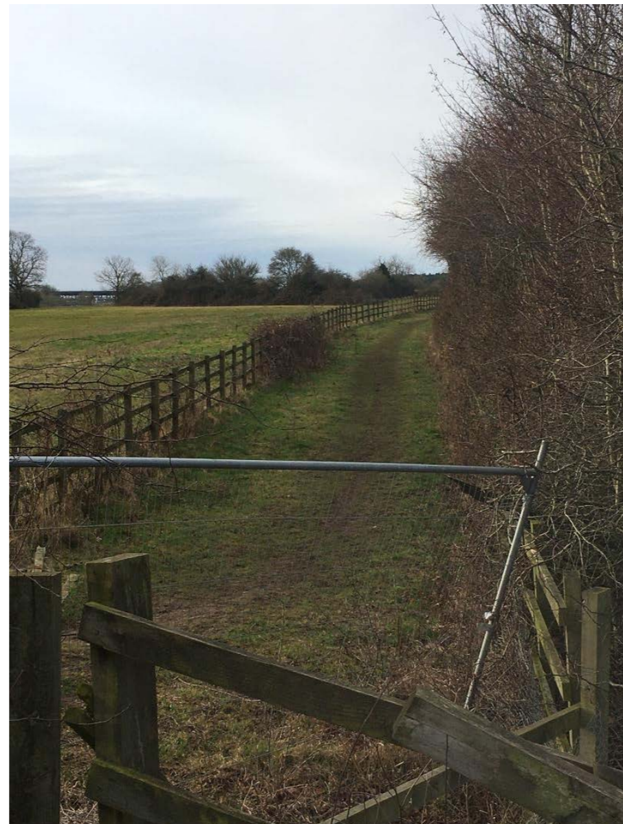
Grassed track requiring resurfacing
