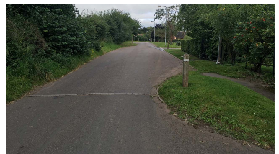
Quiet Lane designations combined with rural traffic calming can encourage slower speeds and courteous behaviour on quiet rural lanes where pedestrians, cyclists and horse riders need to share the space with vehicles
