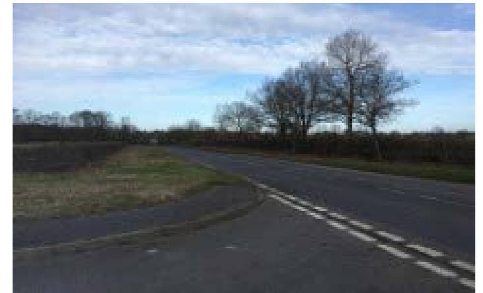
Point at which former A43 crosses B4525
