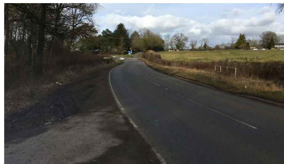
Narrow B4525 is very hazardous for walking and cycling due to HGV traffic
