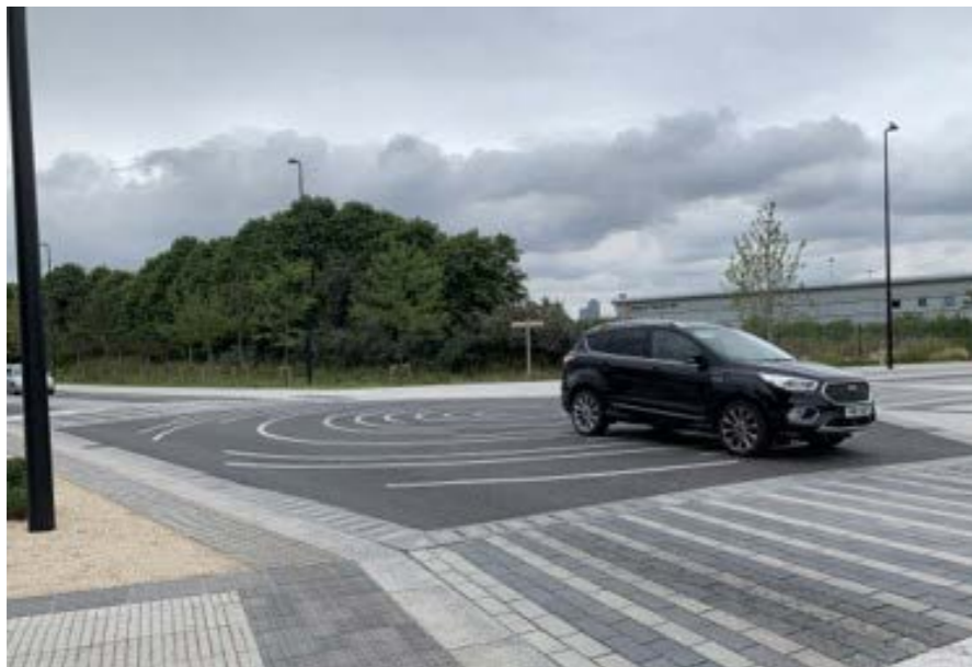
Design measures such as implied roundabouts and zebra crossings can help reduce traffic speeds and encourage drivers to give pedestrians priority (Birkenhead)
