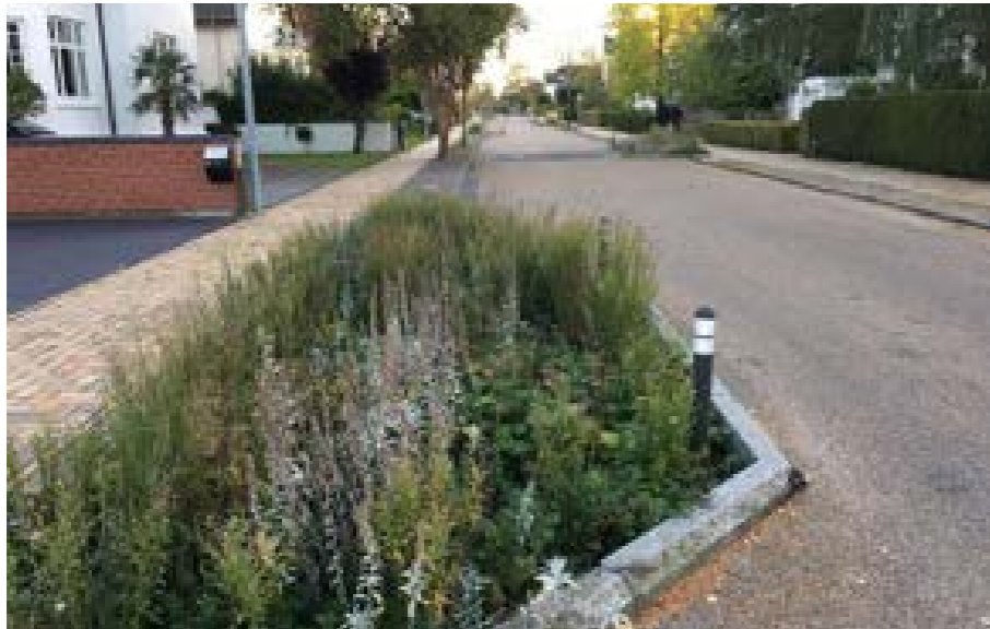
Build outs can provide a sense of arrival and space for planting while having a traffic calming affect
