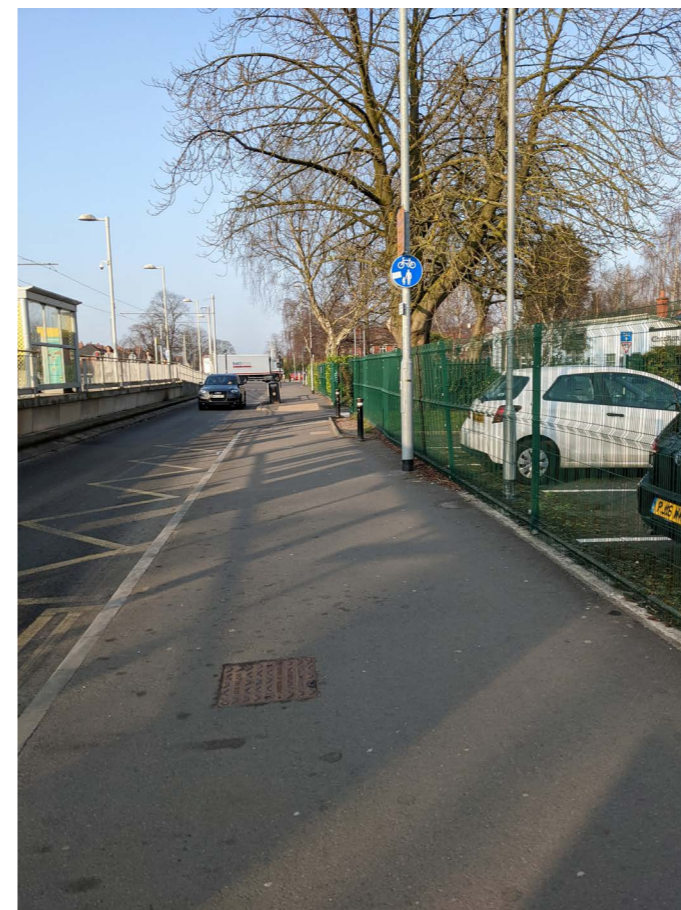
Shared use foot/cycleways can provide a good level of service for both pedestrians and cyclists on rural roads as well as some suburban roads which have few or no active frontages or driveways. A buffer should be provided between the road and the shared use facility on roads with speeds over 30mph.
