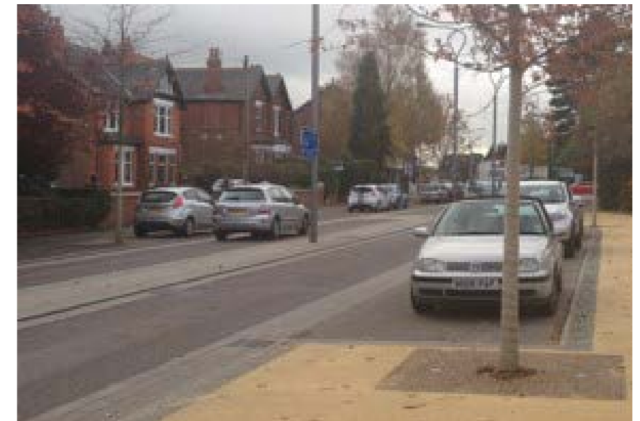
Overly wide carriageways can be put on 'road diets' to reduce traffic speeds and crossing distances. Space for parking can be provided in inset bays so that the carriageway can be kept a consistent width (Poynton)
