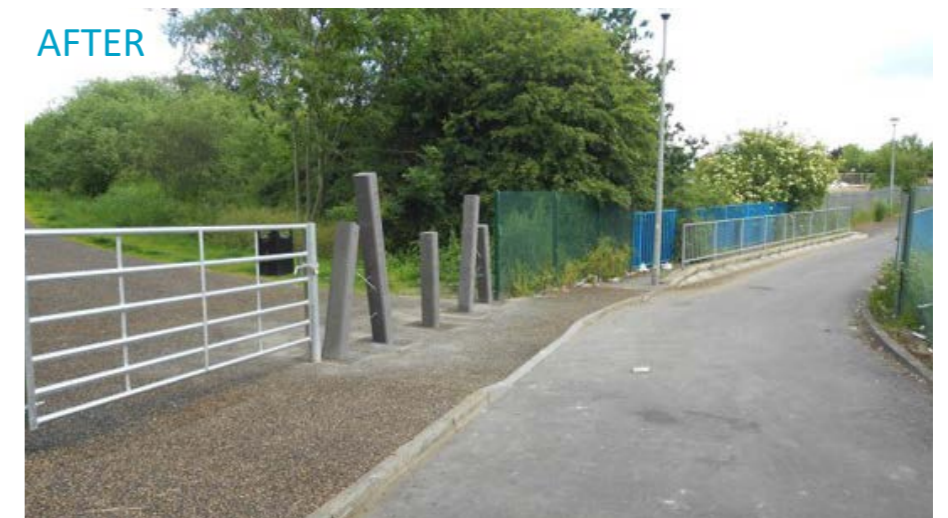
Accessible entrances encourage use by legitimate users including people with wheelchairs, mobility scooters, prams and non-standard cycles (Port Salford Greenway, Salford)
