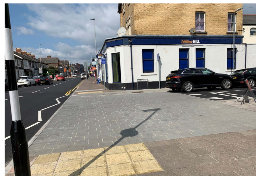
Continuous footways provide priority for pedestrians over cars in areas of high footfall (Cardiff)
