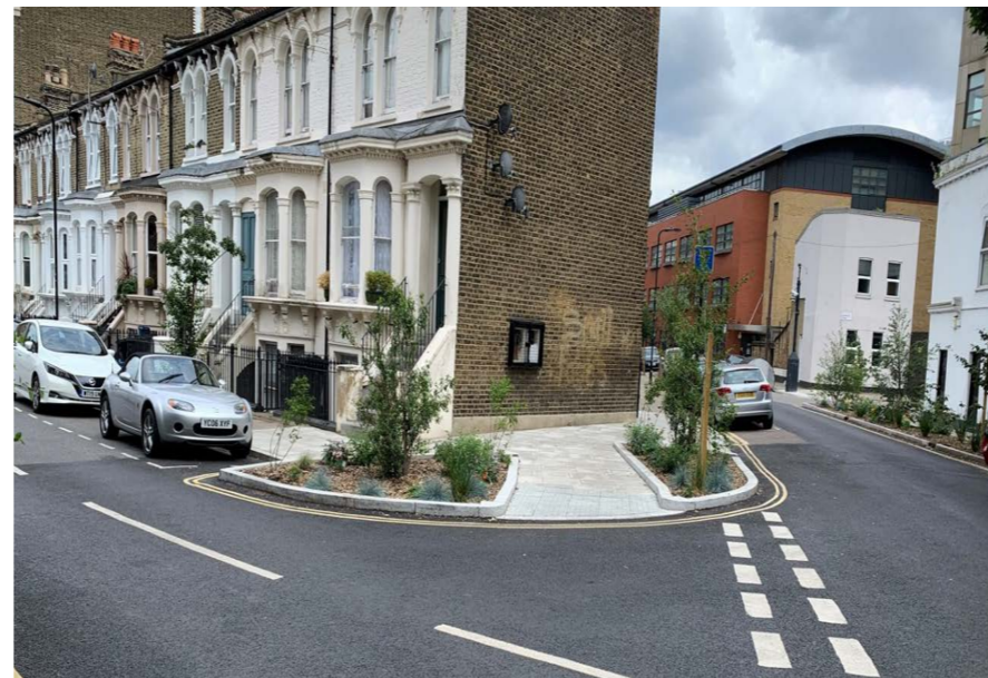
Tightening priority junctions reduces crossing distances and enables crossings to be provided on desire lines. It can also create space for street trees, cycle parking and other street furniture (London)
