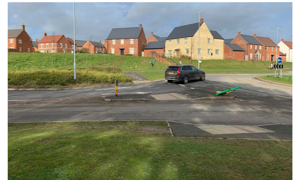
The desire line from the bus stop and Turweston is not currently catered for and crossing facilities at the roundabout near Sainbury's are not sufficient for the volume and speed of traffic
