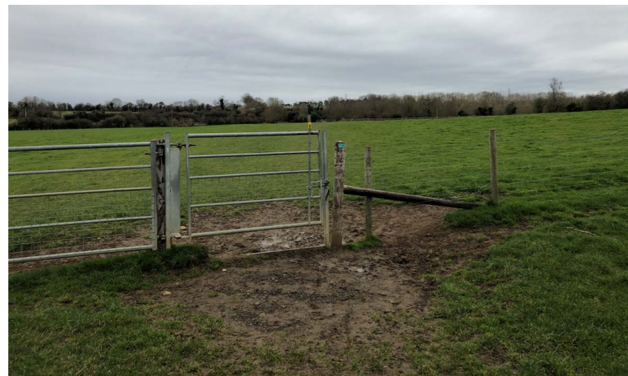
Gates on the route which reduce accessibility
