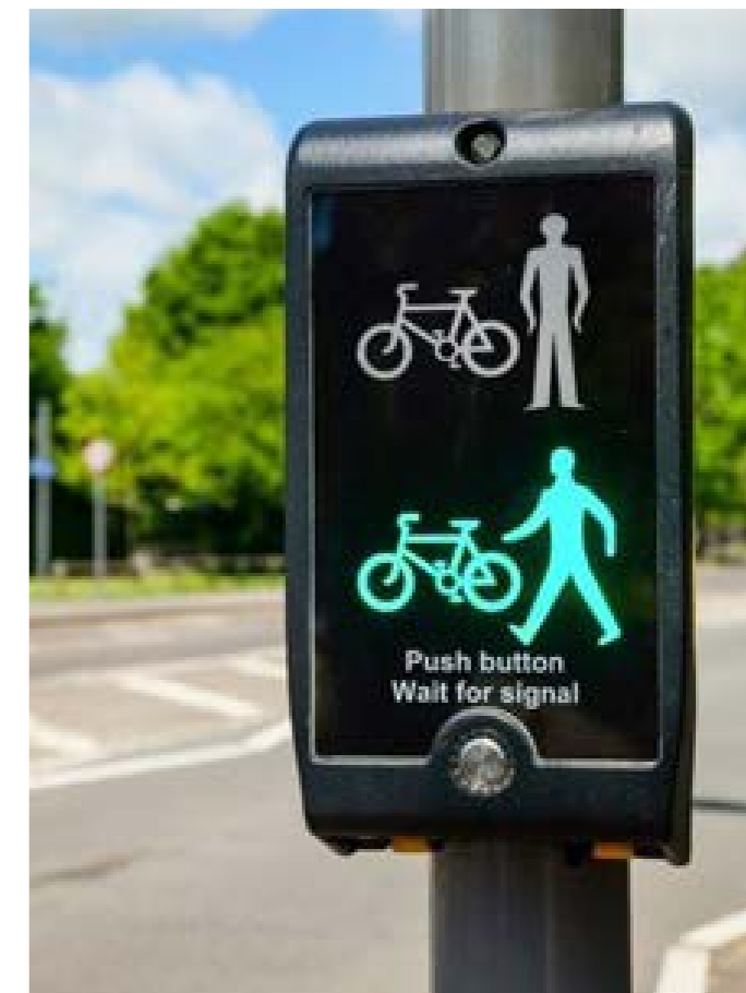
Toucan crossings enable pedestrians and cyclists to cross busy roads and are most suitable where shared provision is provided either side of the crossing.
