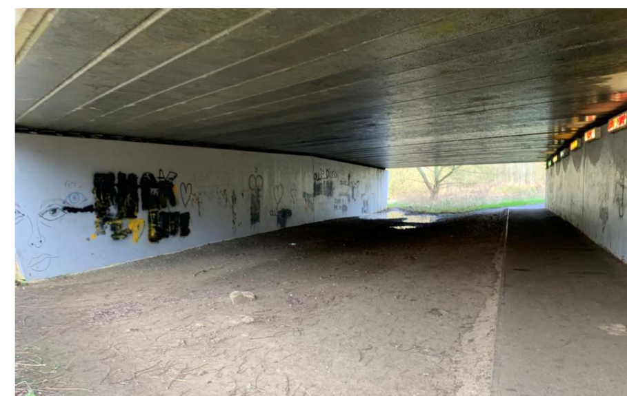
The existing traffic-free route is already well used but is unsurfaced making it very muddy. A sealed surface would ensure it can be used all year-round. The path at the A43 underbridge should be widened to make it more comfortable. Community artwork protected with an anti-graffiti coating could be commissioned to deter anti-social behaviour
