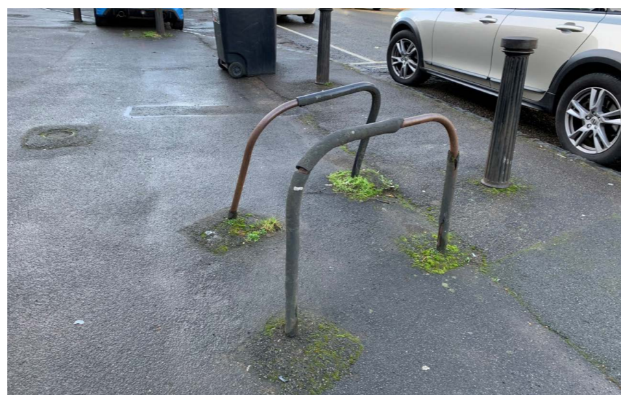
Lack of tactile paving at crossings
