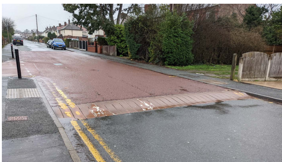
Raised tables and coloured surfacing can act as a gateway feature to slow traffic
