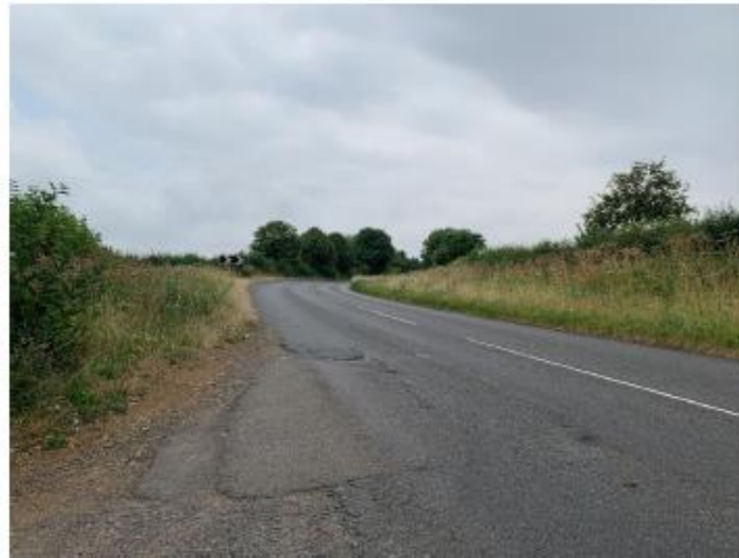
Long Buckby Road is currently National Speed Limit and has no footways or cycling infrastructure.
