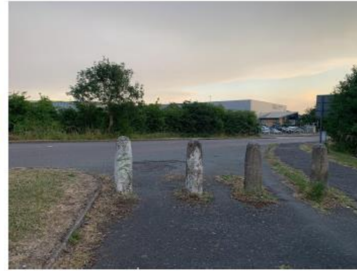
Poor transition between existing facility on the footway and the shared use path under the roundabout via a subway. Inaccessible clearance width between bollards
