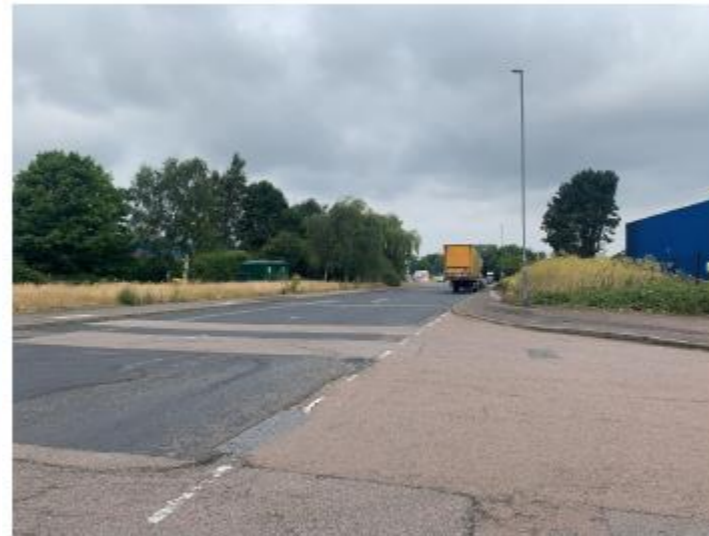
Wide sweeping bends at side roads
