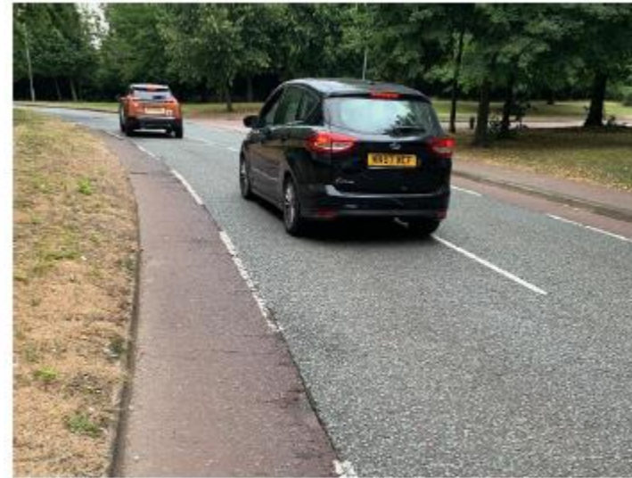
Narrow cycle lanes (in poor condition) and relatively high traffic volumes on Speke Drive create hostile conditions for cycling.
