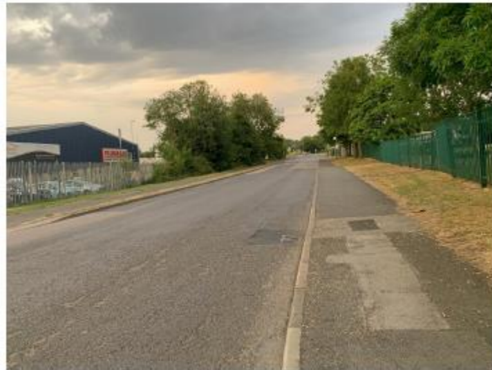
Wide carriageway experiencing higher traffic volumes at peak times. Long, straight geometry facilitates speeding
