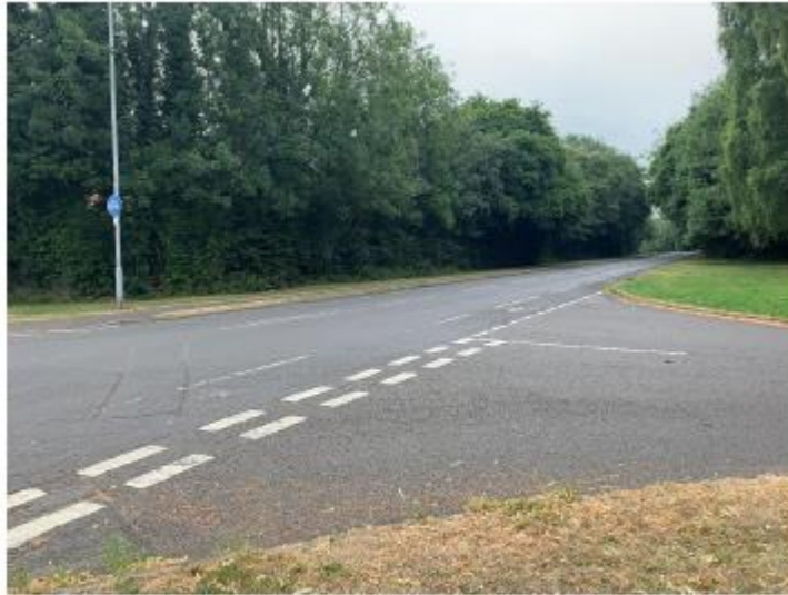
The junction radii at the junctions of Warwick Street and Staverton Road with Western Avenue encourage high traffic speeds and create hostile conditions for cycling in the carriageway.
