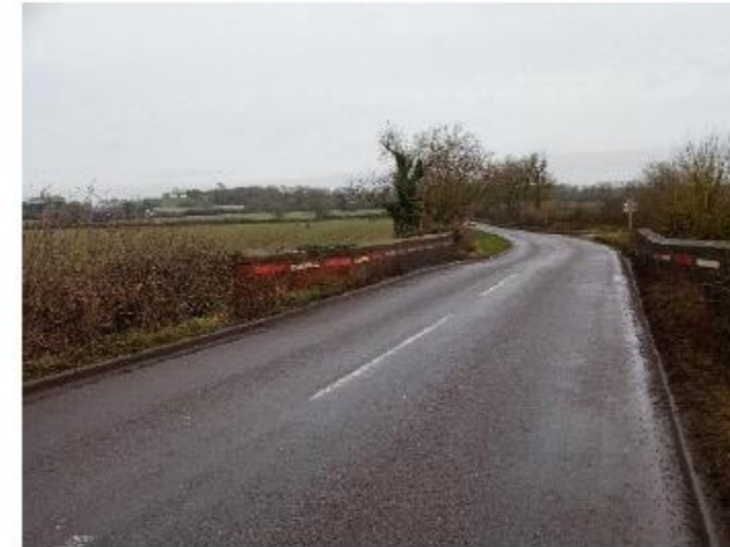
The three Surney bridges on Three Bridges Road create pinch points where there is insufficient space to provide protected space for cycling immediately adjacent to the carriageway.
