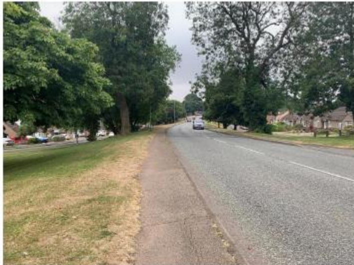
Although there is lots of space and few active frontages along the majority of Ashby Road, the existing footway is narrow with street lighting columns just beyond the back of footway.
