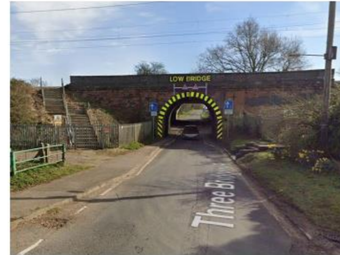
The railway bridge creates a pinch point which narrows the road down to one lane through the bridge.
