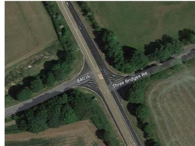
The junction of Long Buckby Road, the A5 and Three Bridges Road is currently very hostile with no crossing facilities for pedestrians and cyclists.
