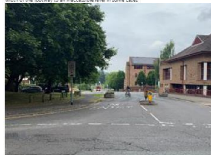
Wide priority junctions put pedestrians in potential conflict with fast turning vehicles and create long crossing distances. They are often excessive for the amount and size of vehicles
