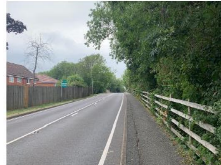
There is a pinch point where Ashby Road crosses over the disused railway line where the total width is less than 8m.
