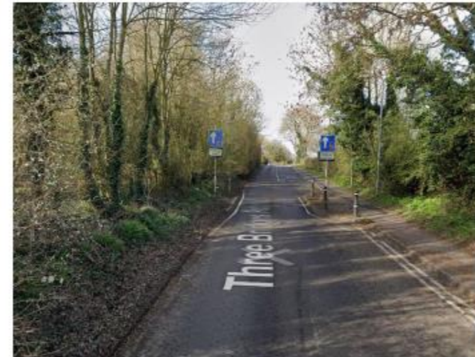
The existing pinch point west of Long Buckby Wharf acts as an effective gateway feature to slow traffic on the approach to the village.
