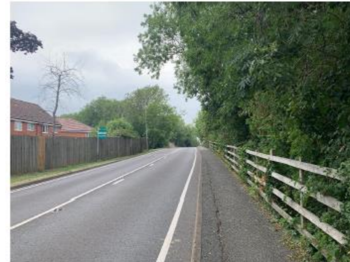
There is a pinch point where Ashby Road crosses over the disused railway line where the total width is less than 8m.
