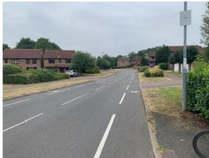
Narrow painted cycle lanes put cyclists in danger of close passes.
