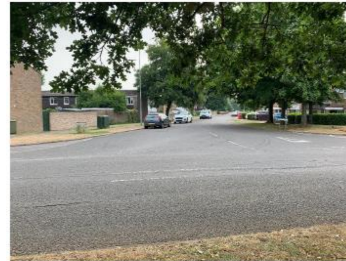
The junction of Staverton Road and Thames Road is excessively wide even with painted hatching to visually narrow the junction. This is likely to encourage higher vehicle speeds and make it difficult for people walking and cycling to cross the road to the bridge.
