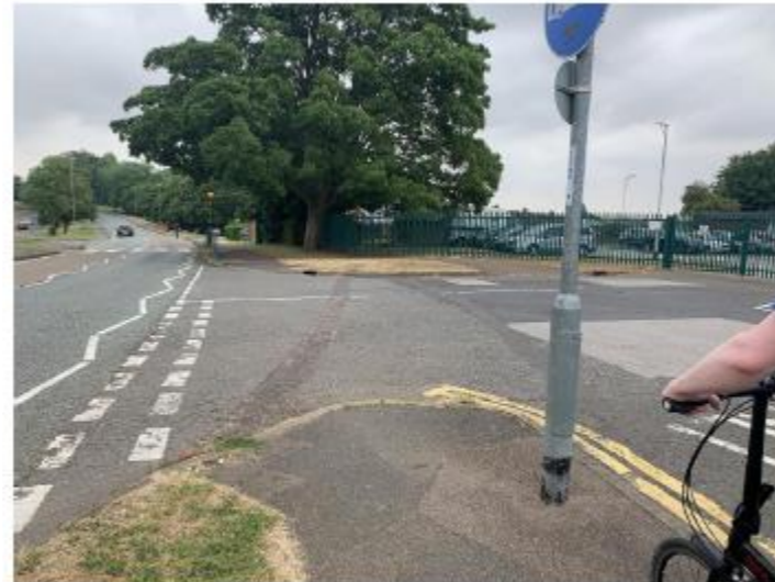
Many of the priority junctions along Ashby Road are very wide with no tactile paving.
