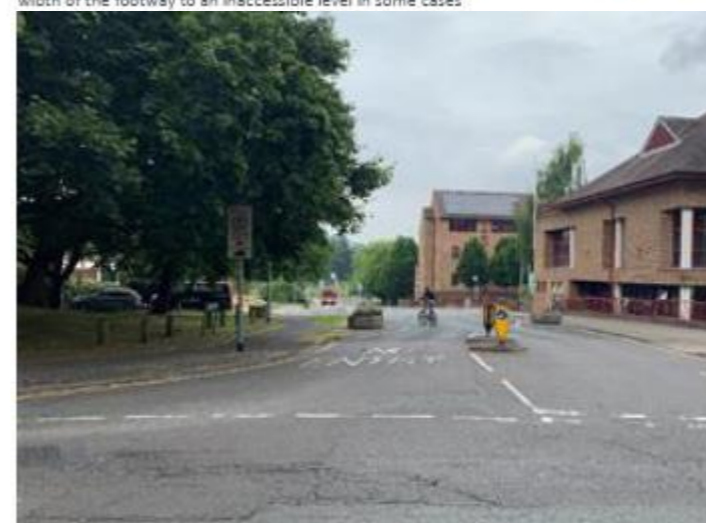
Wide priority junctions put pedestrians in potential conflict with fast turning vehicles and create long crossing distances. They are often excessive for the amount and size of vehicles
