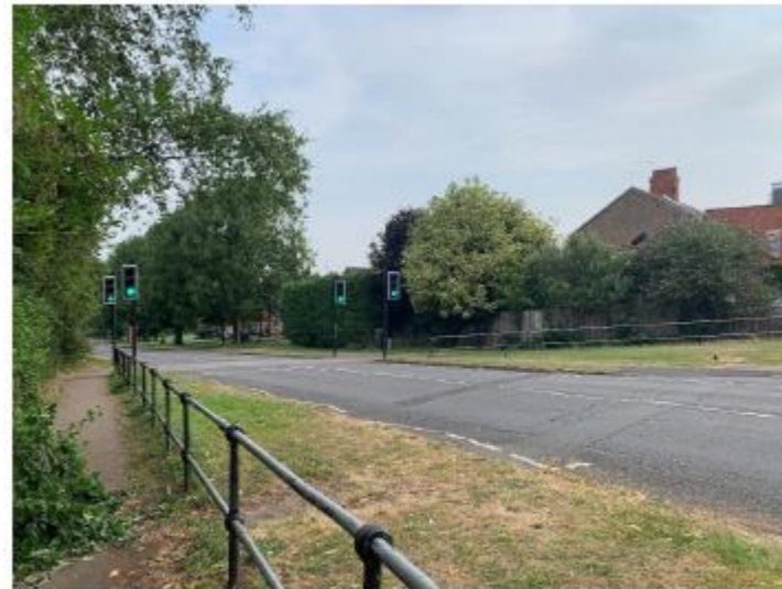
There is an existing Puffin crossing on Western Avenue which takes pedestrians away from the desire line and does not cater for cyclists.
