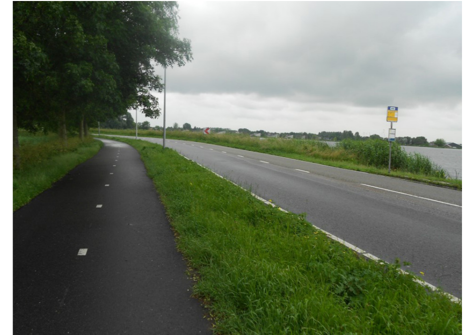
On roads with few active frontages and where roads where pedestrian and/or cycle flows are low, it is often appropriate to provide a two-way cycle track on one side of the road that pedestrians are allowed to use. Priority over side roads should normally be provided.
