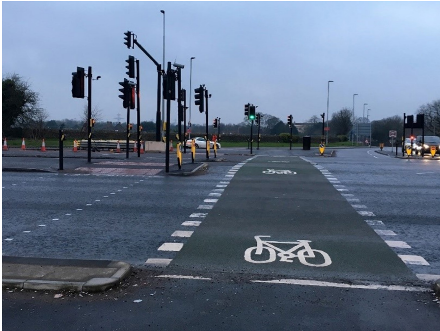
Staggered Toucan crossings are acceptable for locations with low flows of pedestrians and cyclists. However, where there is potential for higher flows, pedestrians and cyclists should be separated at crossings, with a straight across for cyclists at least
