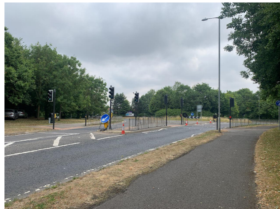
The (staggered) Toucan crossing at the roundabout with Northern Way helps link Drayton Way with new development to the north.
