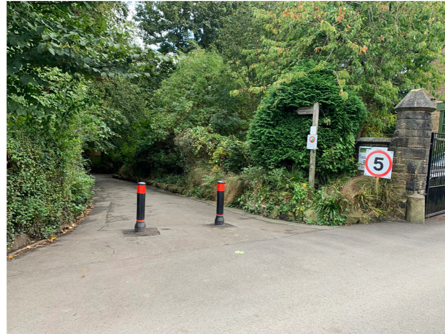
Modal filter should be placed to provide a 1.5m clearance. This will allow access by different types of cycle and ensure accessibility for wheelchair users, those with mobility scooters and those with buggies
