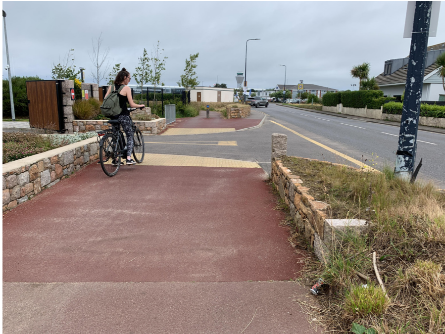
If shared use is opted for, provision should be wide enough to achieve good levels of pedestrian comfort and reduce conflicts. Priority at side roads requires careful consideration
