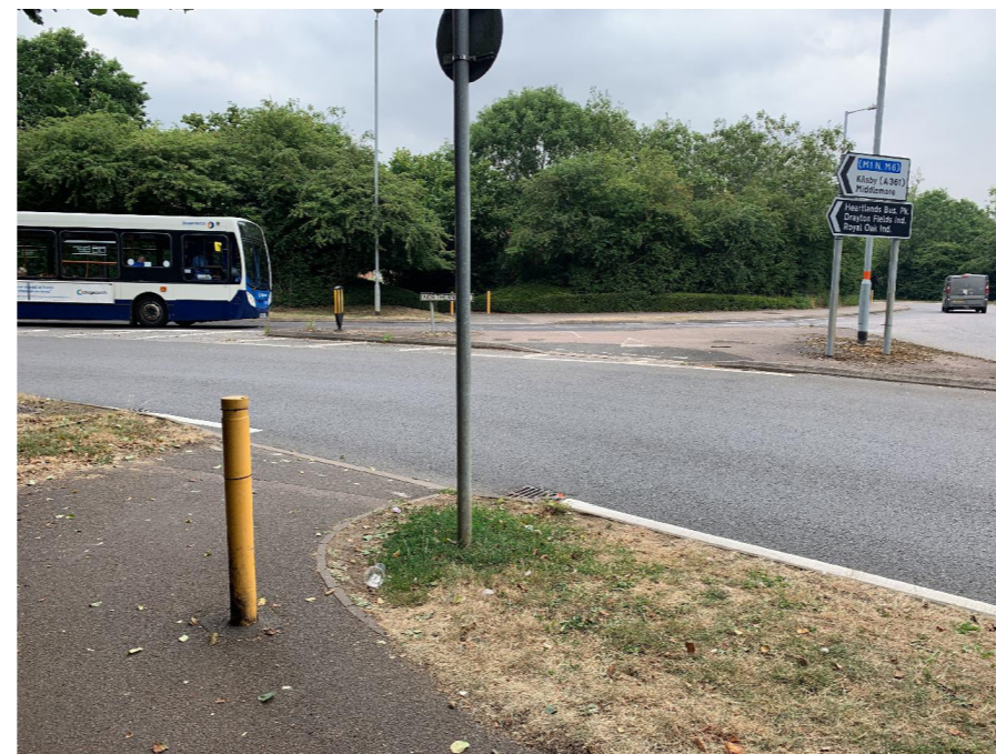
A shared use facility links the end of Speke Drive to the network of shared use paths on Welton Road and Northern Way though signage, transitions and signage is poor.
