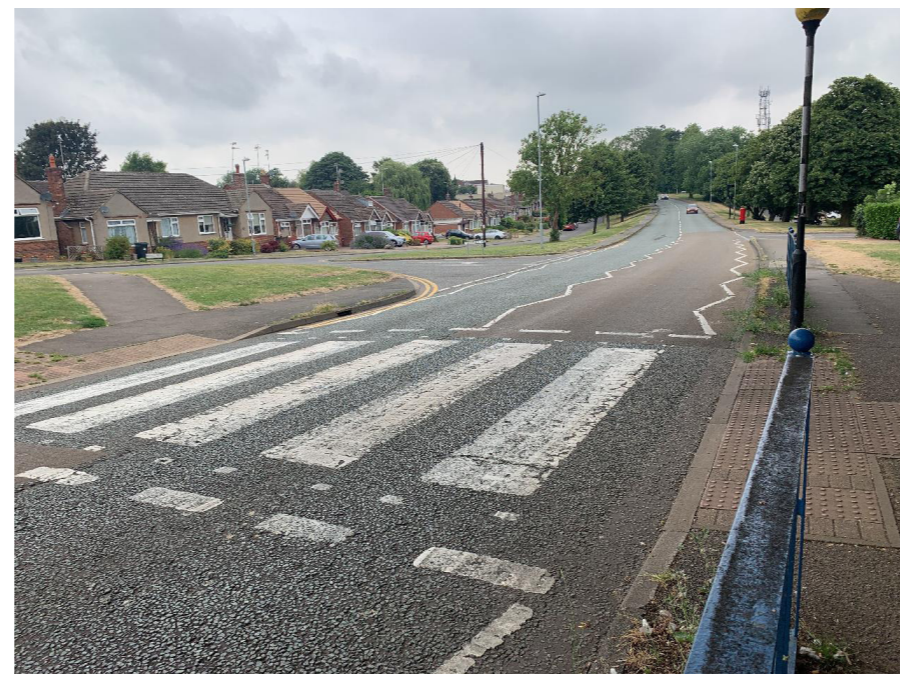
There are existing zebra crossings on Ashby Road but no crossing facilities for cyclists.
