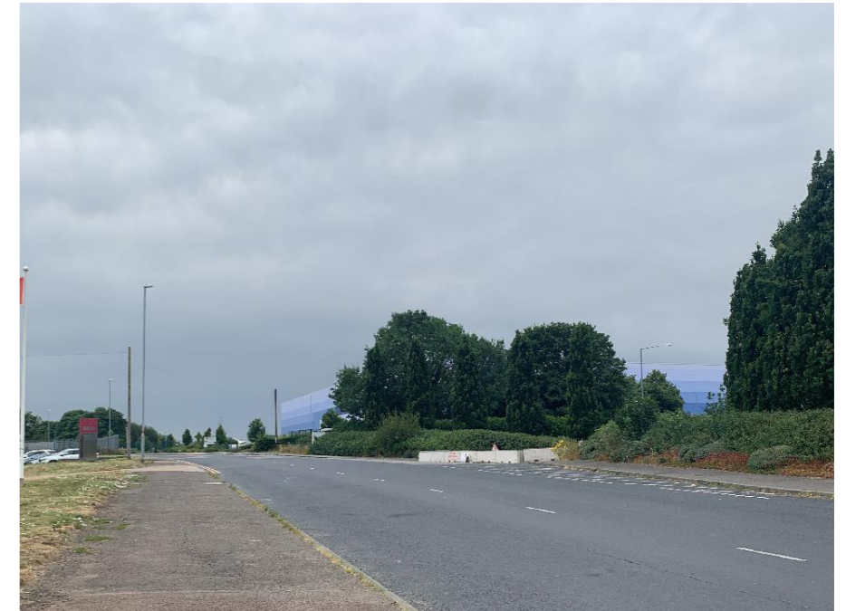
Wide carriageway with hatching, but decent footway provision in terms of width
