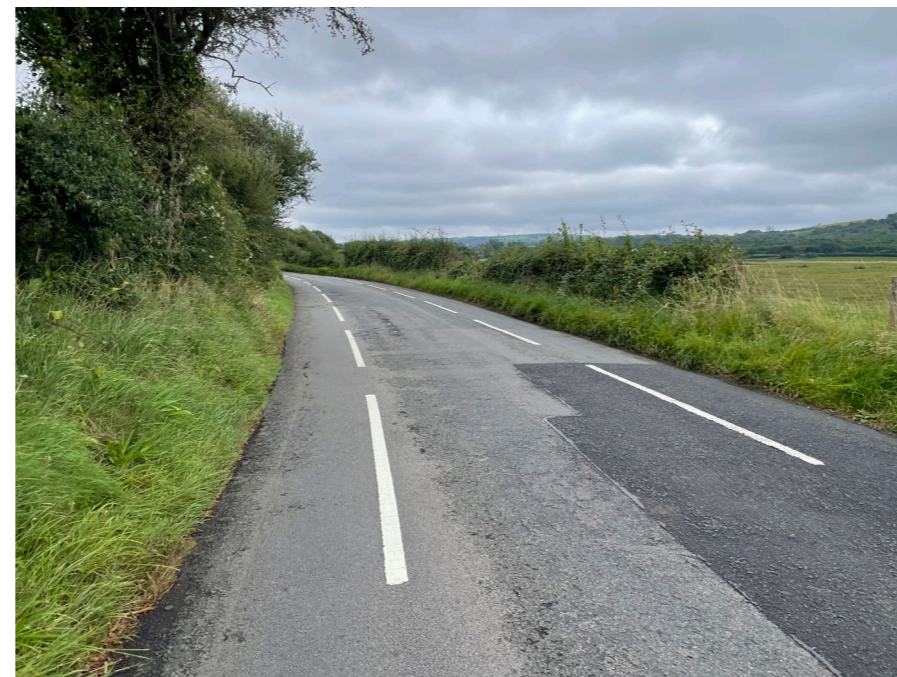
Centre line removal and wide advisory cycle lanes can be a good way of providing cycling infrastructure on more constrained routes where traffic volumes are under 4,000 a day.
