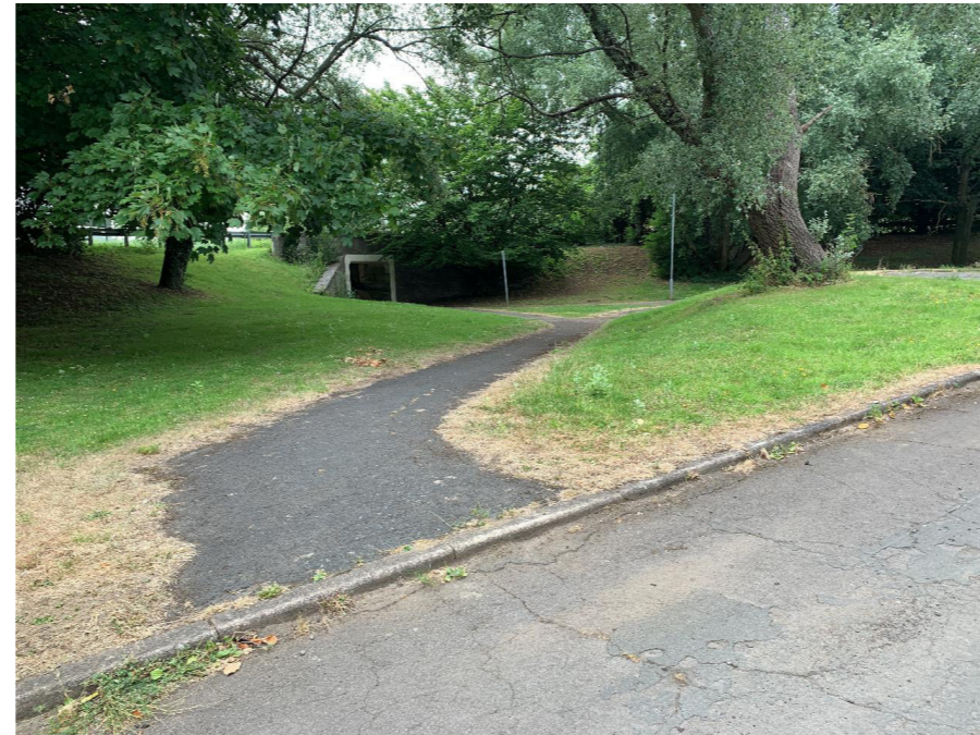
The subway on the north east side of the Eastern Way/Ashby Road roundabout currently only caters for pedestrians and lacks wayfinding.
