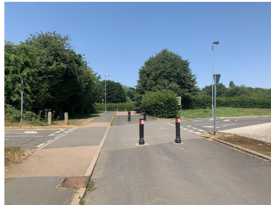
Bollards to the north of the subway ensure motor vehicles are prevented from access the traffic free route while a raised table and continuous footway emphasise that pedestrians and cyclists have priority over drivers accessing the Icon car park (Welton Road, north of Eastern Way).
