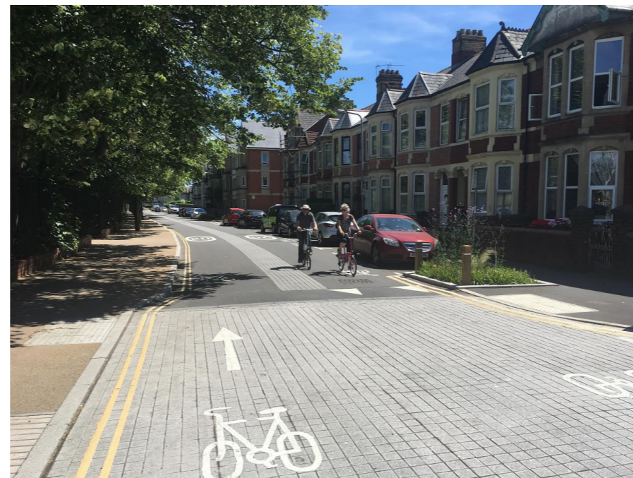
Where there is insufficient space for cycle lanes, traffic calming and visually narrowing can provide a high level of service where traffic speeds and flows are low.
