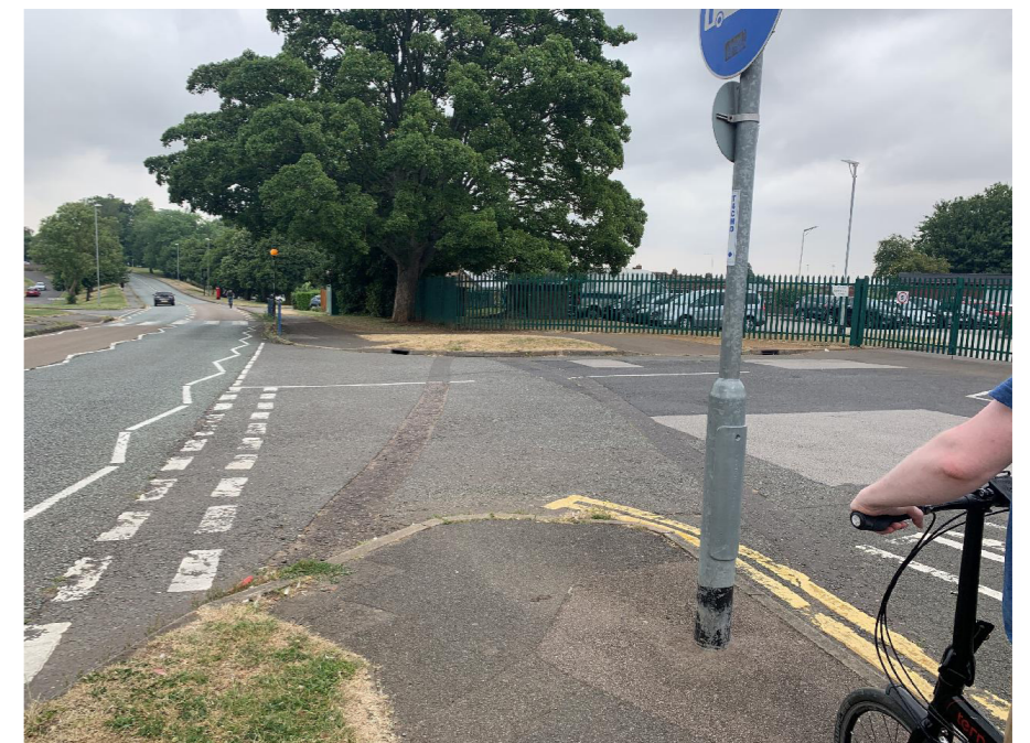
Many of the priority junctions along Ashby Road are very wide with no tactile paving.
