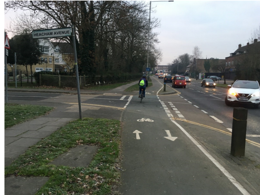
Marked cycle priority should be provided across side roads where possible using give way markings. Bi-directional cycle tracks should be fully or partially set back from the main road and the junction should be tightened as much as possible to slow turning vehicles.
