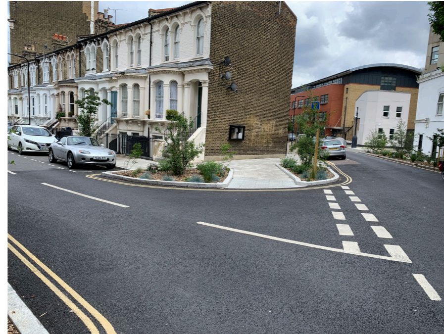
Tightening up priority junctions reduces crossing distances for pedestrians and slows turning vehicles. It can also provide space for greening, where needed.
