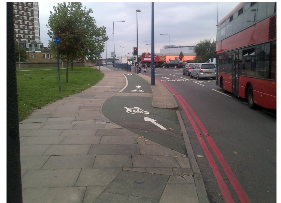
Clear transitions should be provided where cyclists need to leave or join the carriageway, for example to reach a crossing or transition to a cycle track or shared use facility.
