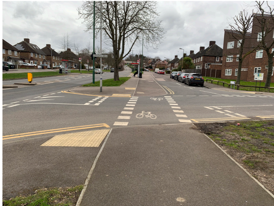
Where cycle tracks or footways meet priority junctions, generally implied or designed priority should be provided for cyclists and pedestrians
