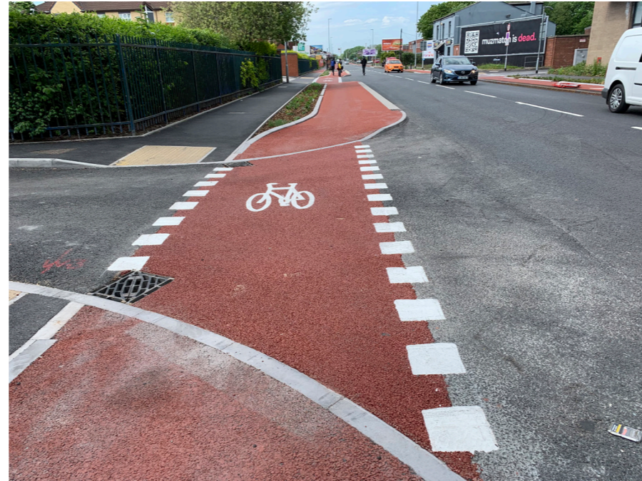
Priority at side roads can be successfully created using continuous markings in visible colours. Setting the crossing back over side roads can also help to improve visibility
