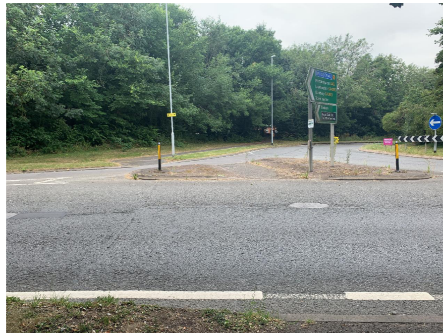
The lack of controlled crossings at the western end of the route limits its utility value, particularly the lack of crossing over the southern arm would enable a strong connection through to Riley Close and the Royal Oak Industrial Estate.
