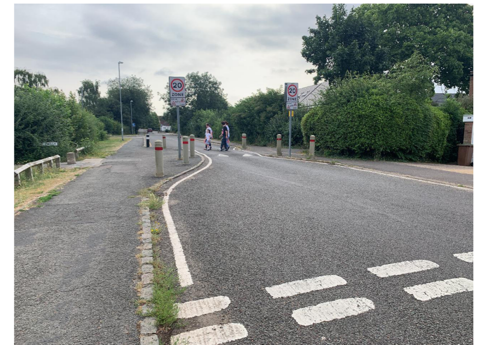
Priority pinch points can slow vehicle speeds and discourage unnecessary through traffic on routes. They can be particularly effective when they include a cycle bypass.
