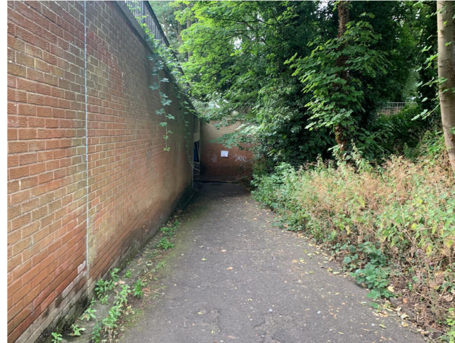
Poor sight lines negatively impact on the feeling of personal safety and encourage people to crossing the road rather than use the subway (Yeomanry Way/Staverton Road).
