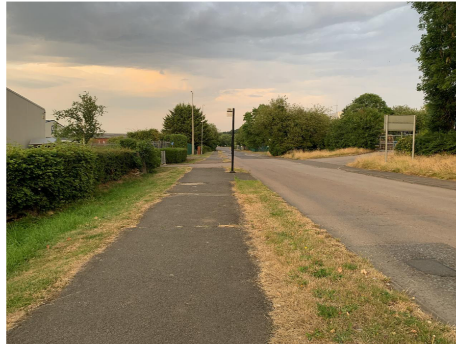
Existing wide footway which could provide a shared use path of widened/resurfaced
