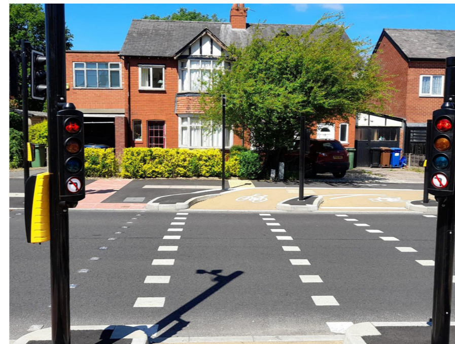
Signalised parallel crossings can be used in environments with higher traffic speed and volumes, providing priority and full separation for pedestrians and cyclists
