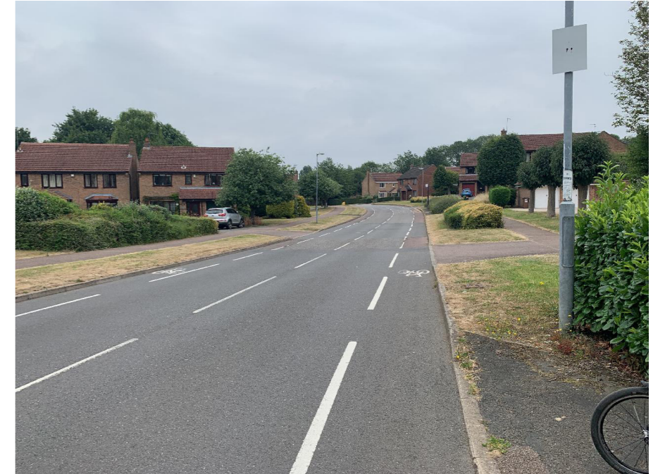
Narrow painted cycle lanes put cyclists in danger of close passes.
