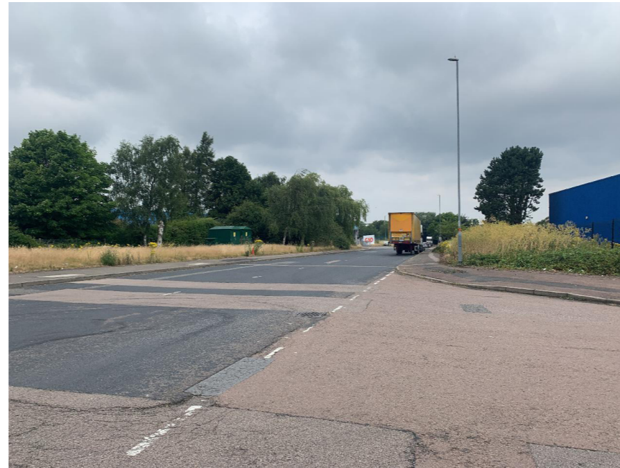
Wide sweeping bends at side roads
