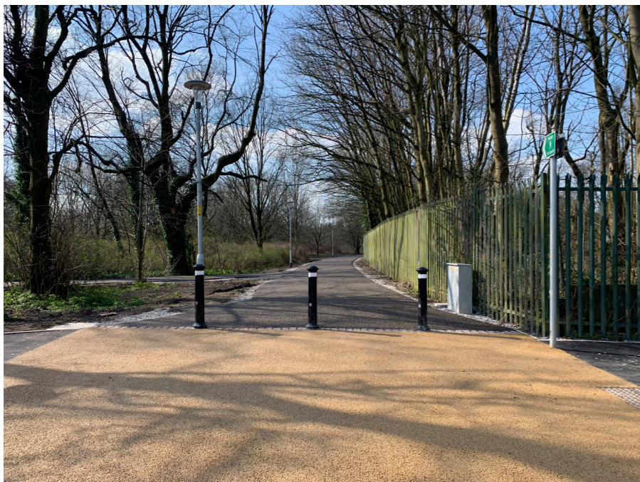
Transitions from the protected facility on Long March to the off-road shared path needs to be smooth and obvious. Bollard spaces should be 1.5m minimum to ensure access for all
