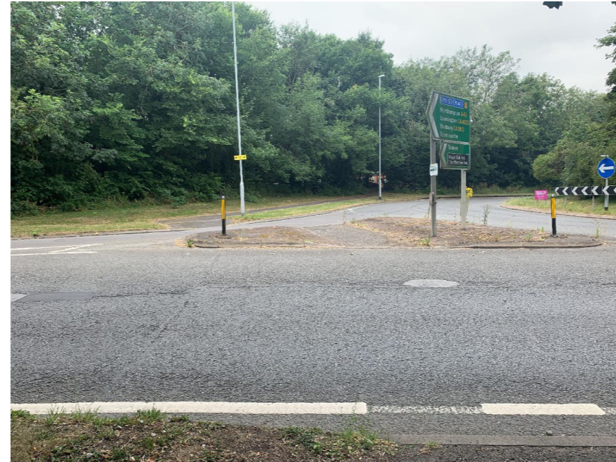
Uncontrolled crossing point on the A361/A45 roundabout on a pedestrian and cycle desire line on the existing shared use footway/cycleway. The wide carriageway and proximity to the roundabout make it difficult for pedestrians and cyclists to judge when it is safe to cross.
