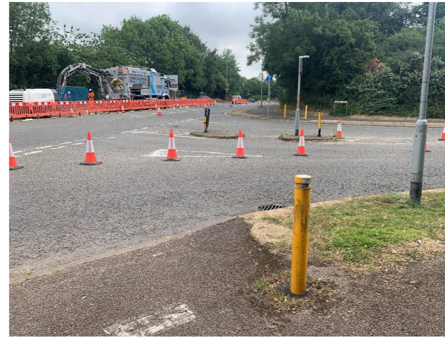
The junction of Ashby Road and Drayton Way is currently a wide priority junction which is hazardous for pedestrians and cyclists.
