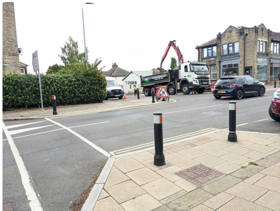
Raised tables and build outs can be used to create implied crossing points and to slow traffic
