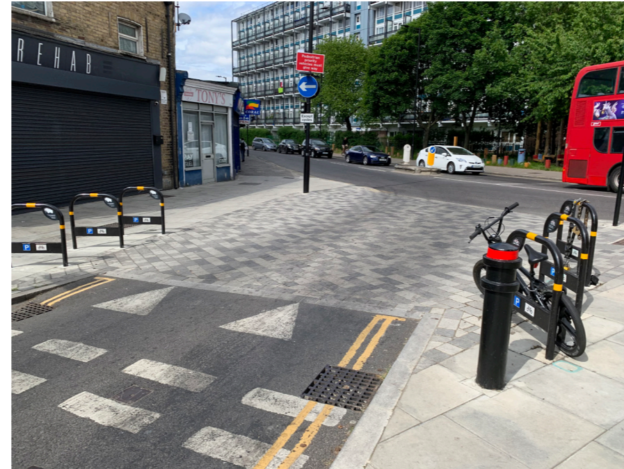
Where traffic flows are low, continuous footways can be provided over side roads to reinforce pedestrian priority. This is particularly useful where there are higher pedestrian flows, such as near to shops or schools
