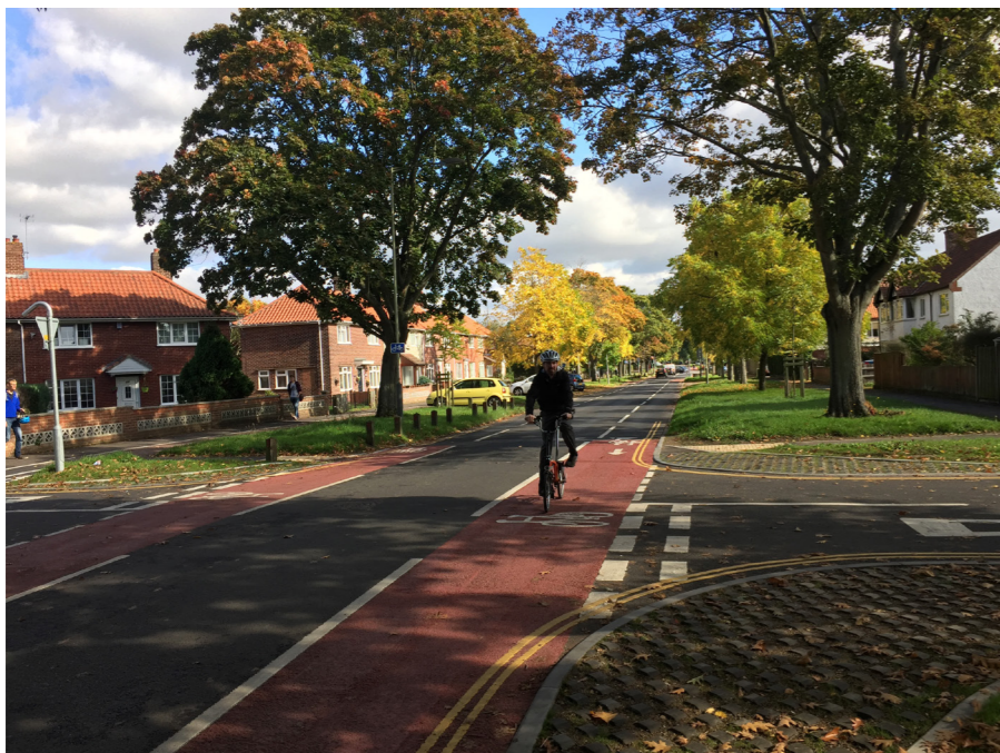
Wide advisory cycle lanes and centre line removal can reduce traffic speeds and provide a good level of service where narrow carriageway widths would not otherwise enable the introduction of cycle lanes.
