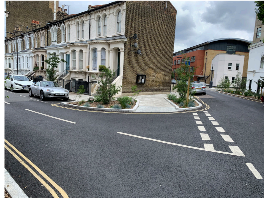
Narrowing priority junctions and overly wide carriageways can help calm traffic as well as providing space for wider footways and greening.
