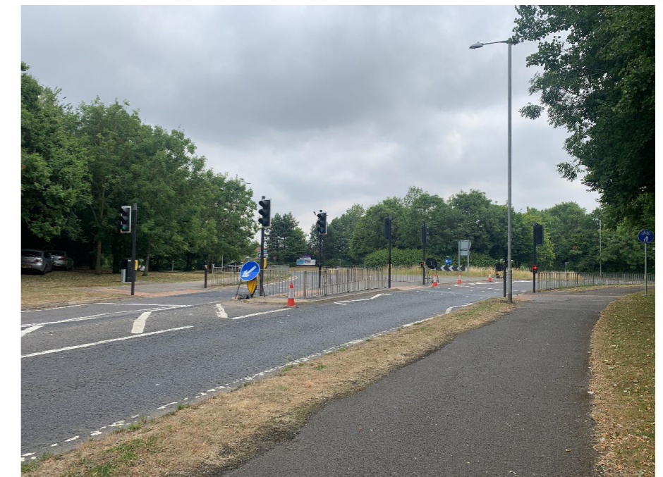
An existing staggered Toucan crossing on Drayton Way caters for pedestrians and cyclists travelling north-south but all other arms of the roundabout are uncontrolled (Drayton Way/Northern Way).
