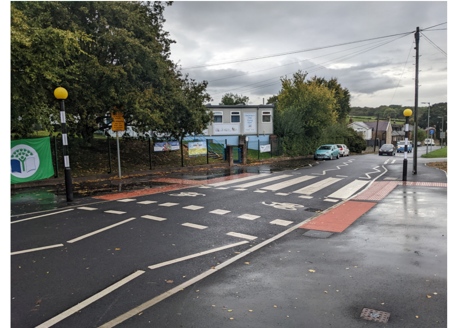
Parallel crossings provide safe crossing points whilst keeping pedestrians and cyclists separate, such as this example near a school in North Wales
