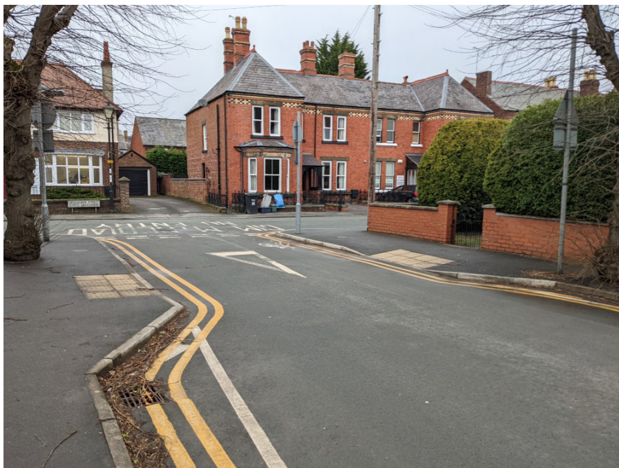
Narrowing priority junctions can include making side roads entry/exit-only, creating short distances for pedestrians to cross and requiring drivers to turn carefully
