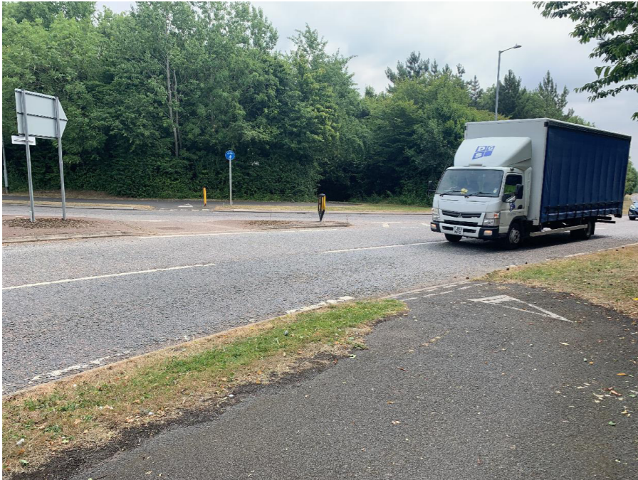
Uncontrolled crossing of the southern roundabout arm with give way markings on the shared footway/cycleway mean pedestrians and cyclists have to wait for a gap and cross two lanes of traffic to get to the refuge (Drayton Way/Northern Way)
