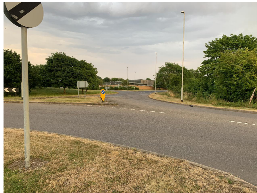
Route ends at roundabout where cyclists are kept on a shared path away from the carriageway
