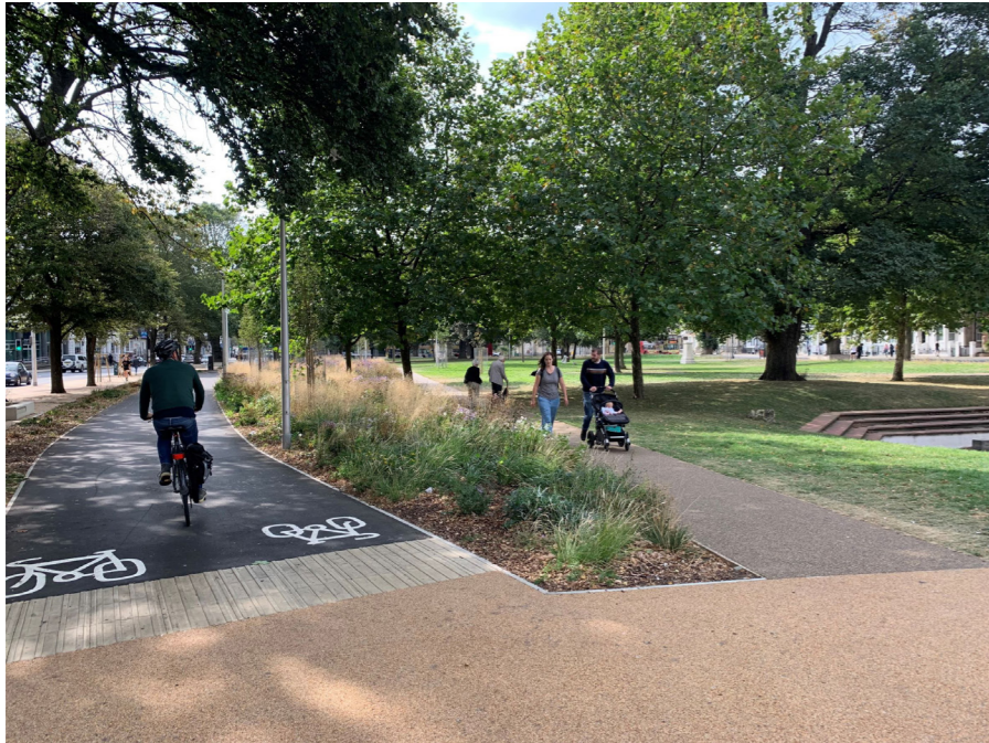
Where there are higher flows of pedestrians and/or cyclists and where space allows providing separate facilities for pedestrians and cyclists can reduce conflict and increase the sense of comfort.
