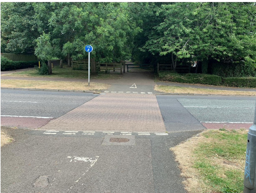
Design priority for pedestrians and cyclists through the use of block paving is compromised by give ways on the shared use path which could cause confusion about who has priority (Shackleton Drive/disused railway line).
