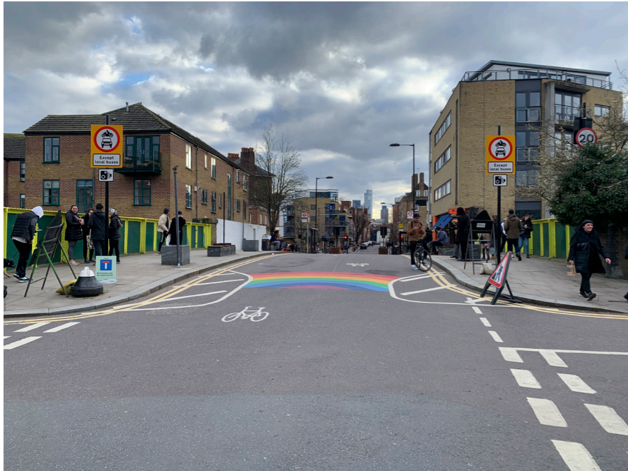
Bus gates are a good way to prevent rat running to reduce traffic flows and enable cycling in mixed traffic streets while maintaining bus routes and access to homes.
