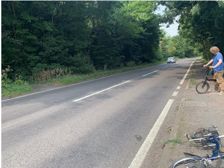
This uncontrolled crossing point is difficult for motorists to spot and is located just west of where the A45 changes from 40mph to National Speed Limit, making it very difficult for pedestrians and cyclists to cross (A45 Braunston Road).
