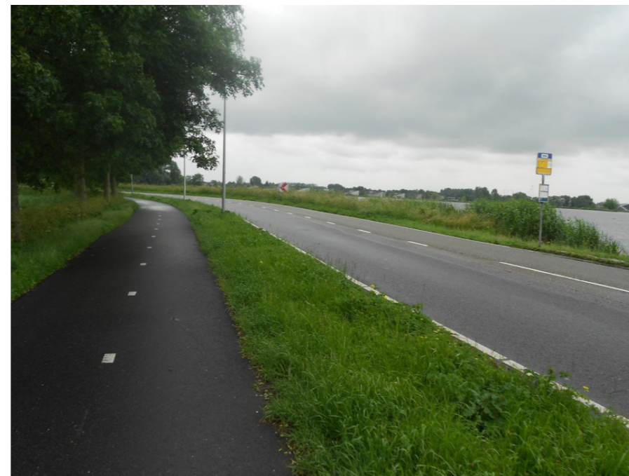
Even where shared with low numbers of pedestrians, it is important to design facilities to meet the needs of cycle traffic. Providing a centre line helps remind pedestrians and drivers to expect cyclists and encourages pedestrians to walk on the left.
