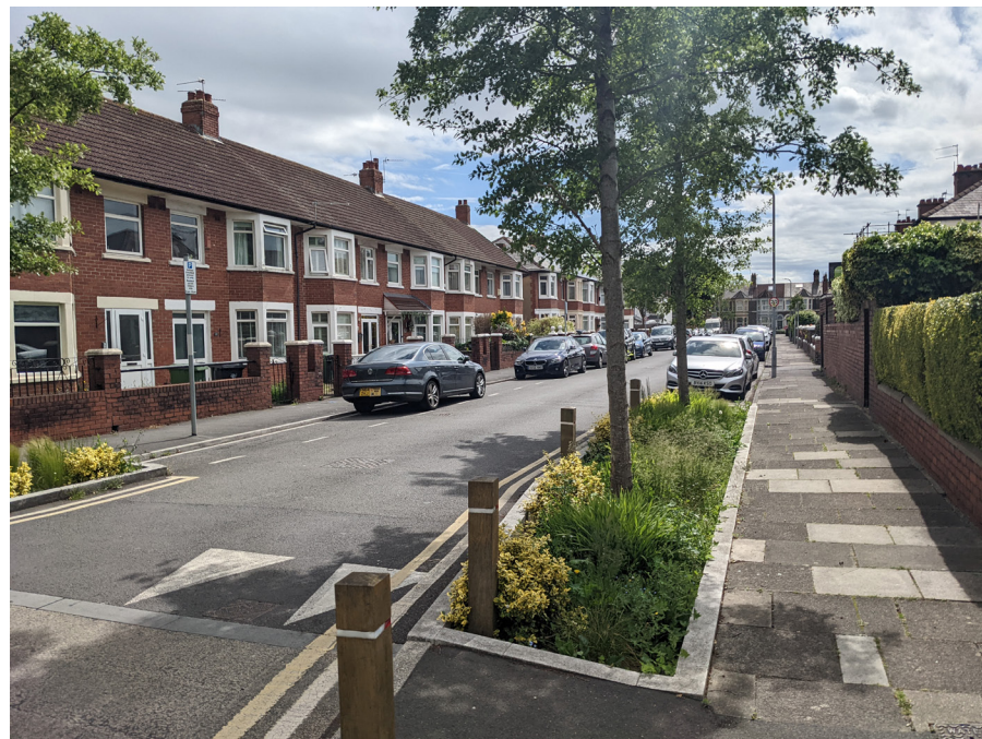
Footway build outs provide an opportunity for greenery and water retention, which can help to reduce pooling in the carriageway and on the footway
