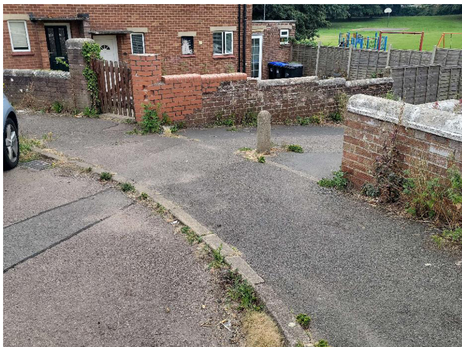
Some entrances to traffic-free routes are missing dropped kerbs and tactile paving entirely. This would likely require supporting parking restriction measures.
