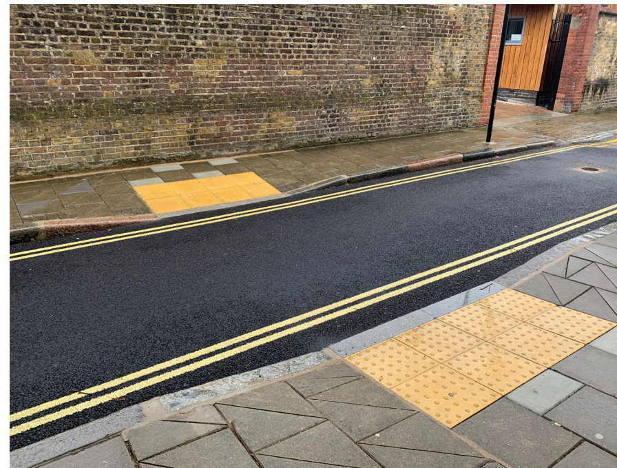
Informal crossing points should be used to supplement formal crossing points in order to meet pedestrian desire lines. They should have dropped kerbs flush to the carriageway with correct use of tactile paving
