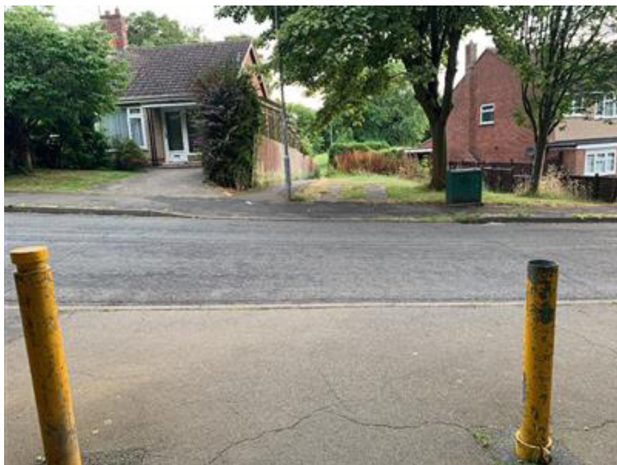
Connections between some traffic-free paths lack dropped kerbs and tactiles, making them less user-friendly for those who are partially sighted or unable to bump down kerbs
