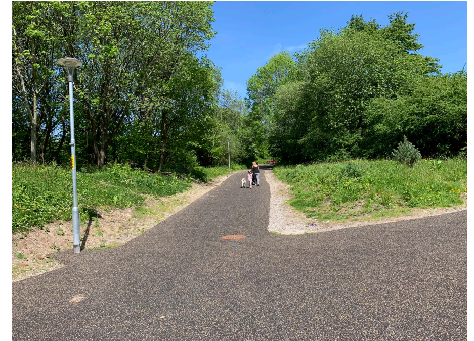
Traffic-free routes should be wide and smooth, allowing comfortable access for those with wheelchairs or buggies. Lighting should be included to ensure year-round use
