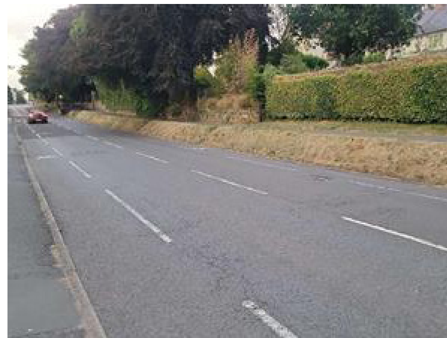
Level differences between the footway and the carriageway reduce the ability for pedestrians to cross informally
