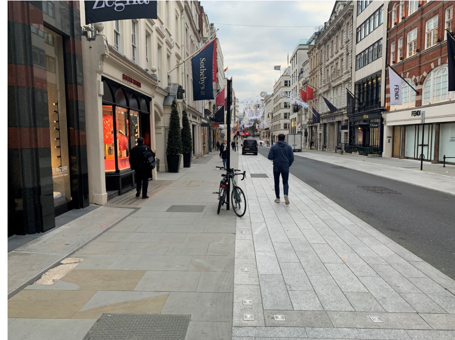
Flush parking bays can effectively widen the footway, providing additional space for walking when not in use for parking or loading.
