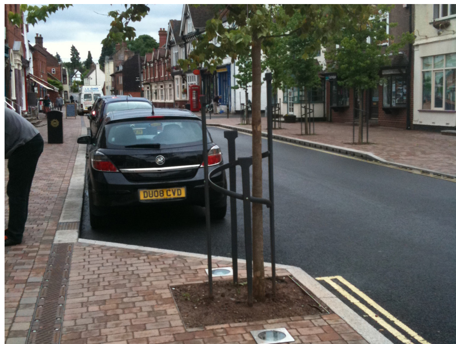
Formalising parking helps to visually narrow the carriageway and slow down drivers, but also allows for build outs between parking spaces, on which street furniture or greenery can be provided
