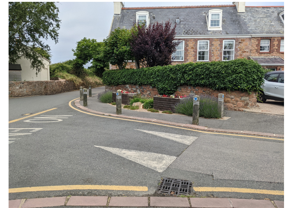
Raised tables over junctions can act as traffic calming whilst also providing an informal crossing point which is flush to the kerb. This can be particularly useful for those with wheelchairs or buggies. Creating these in different colours can increase their effectiveness.
