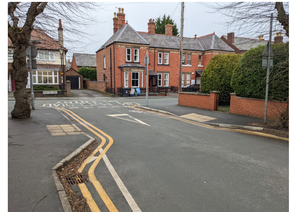
Narrowing priority junctions and building the footway out helps to create safer and easier crossing points for pedestrians whilst also encourage drivers to turn in and out with more care
