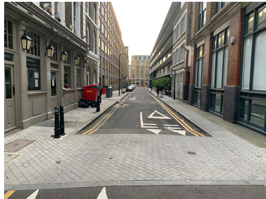
Continuous footways over side roads helps to physically reinforce pedestrian priority over turning vehicles. They can improve pedestrian comfort by offering a flush crossing point
