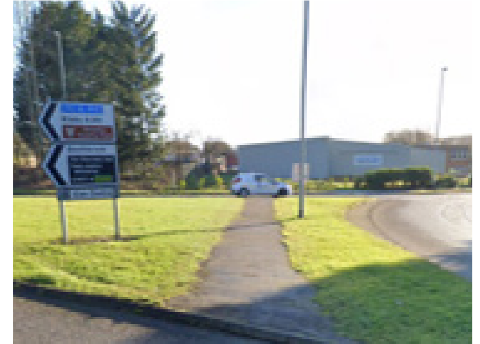
There are currently no crossing facilities – not even dropped kerbs – at the London Rd/A425/ Stefen Way roundabout.
