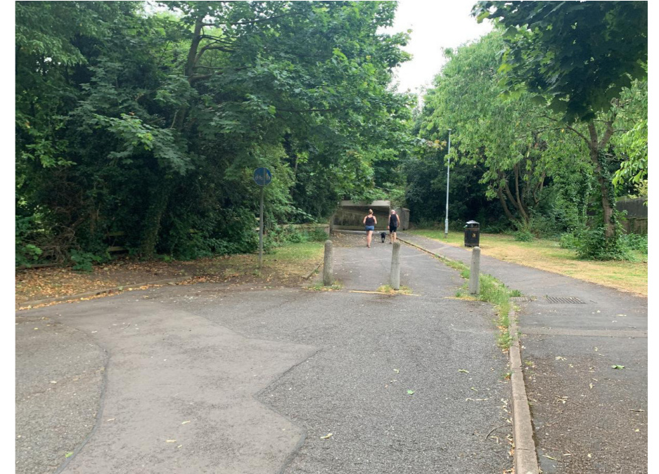
The subway between Abbey Street and Norton Road under the A425 is well maintained and was observed to be well used.
