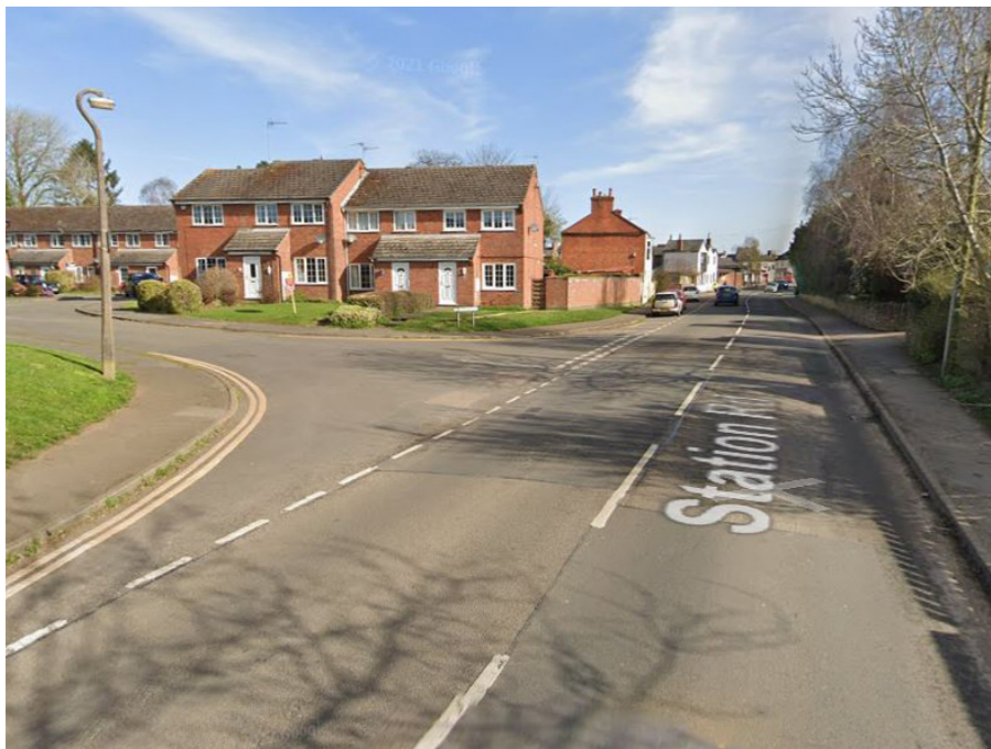
Some priority junctions along Station Road have very wide radii, creating long crossing distances for pedestrians and increasing the risk of left and right hooks for cyclists in the carriageway from turning drivers.
