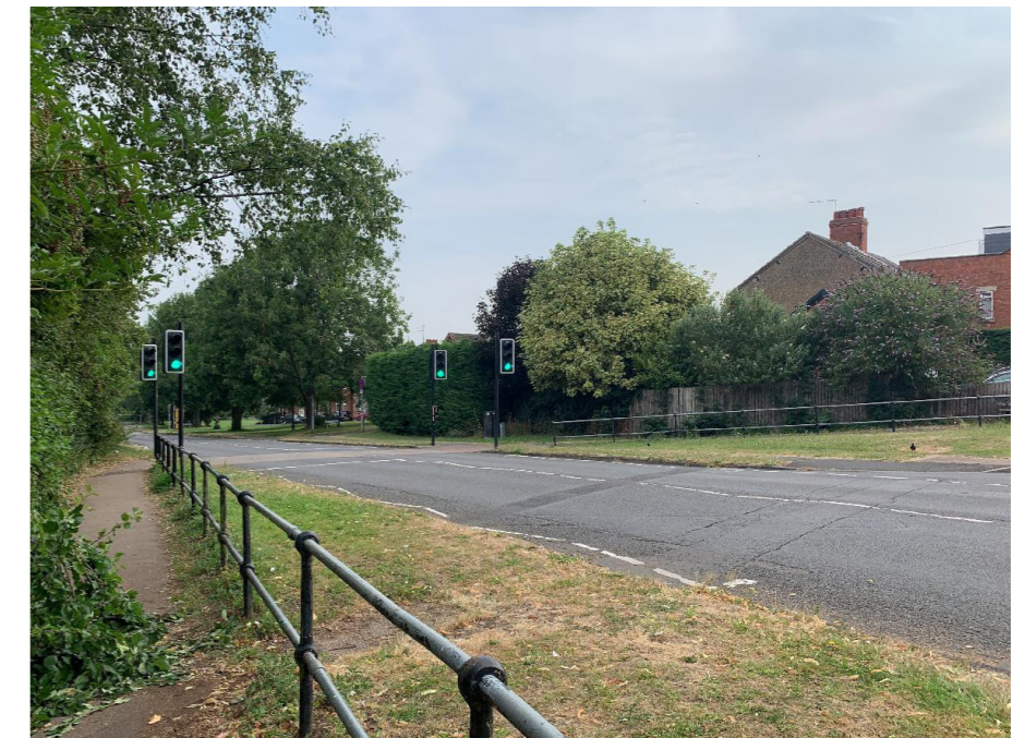
There is an existing Puffin crossing on Western Avenue which takes pedestrians away from the desire line and does not cater for cyclists.
