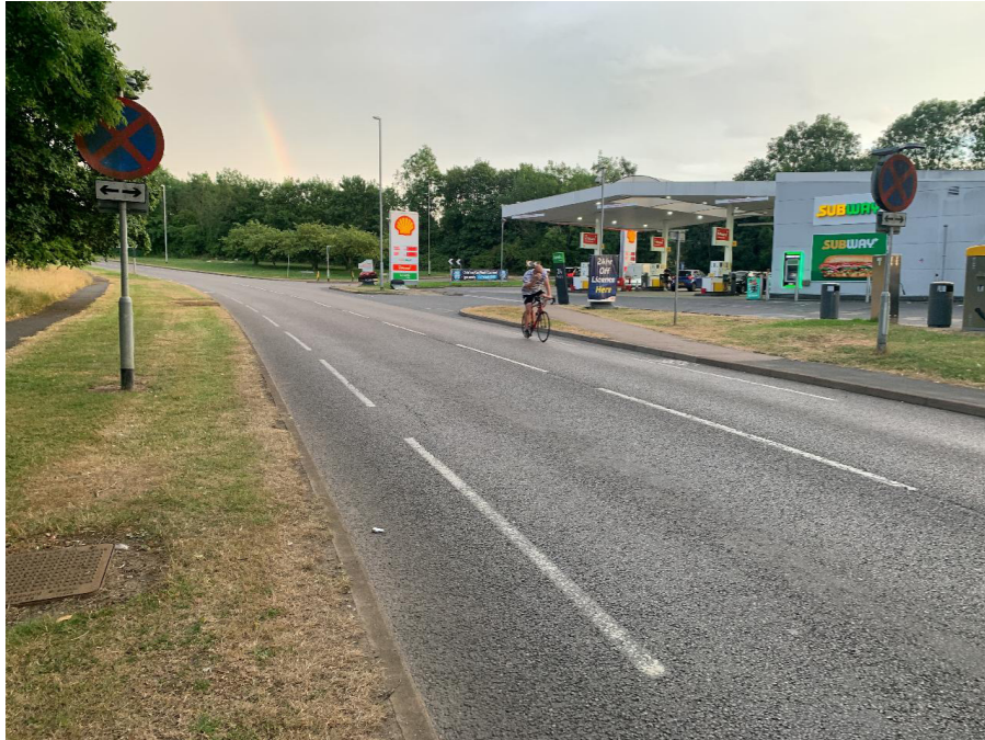
Narrow painted advisory cycle lanes are inappropriate on routes with traffic volumes above 5,000 and speeds above 20mph.
