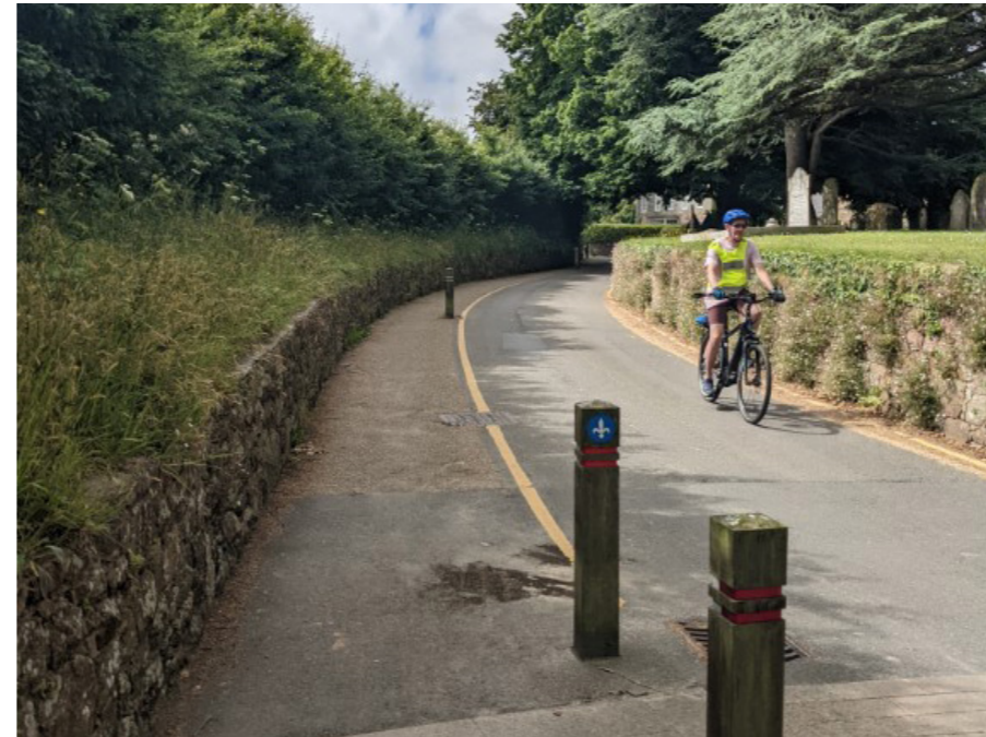
Implied footways with passing places for cars provide protected space for walking and can significantly reduce speeds as well as flows by making routes less attractive for vehicles
