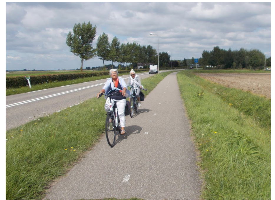
On rural roads where pedestrian and cycle flows are very low, it is often appropriate to provide a two-way cycle track on one side of the road that pedestrians (and horse riders) are allowed to use. Priority over side roads should be provided wherever safe to do so.
