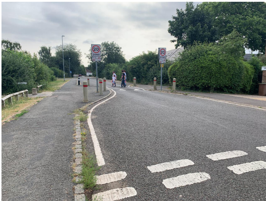
Staverton Road is relatively wide and straight which may encourage high vehicle speeds. However, the 20mph zone and priority pinch points with raised tables appear to work well with drivers generally giving way to pedestrians crossing.
