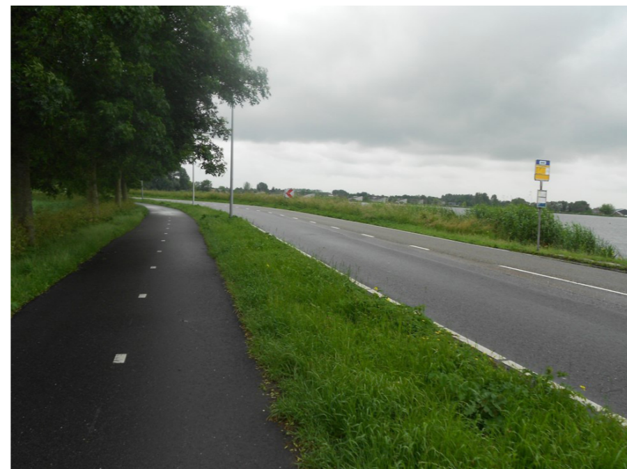
Cycle tracks that are designed for low flows of pedestrians and horse riders to share can provide a good level of service for all users on rural roads which have few or no active frontages or driveways. A buffer should be provided between the road and the shared use facility on roads with speeds over 30mph.
