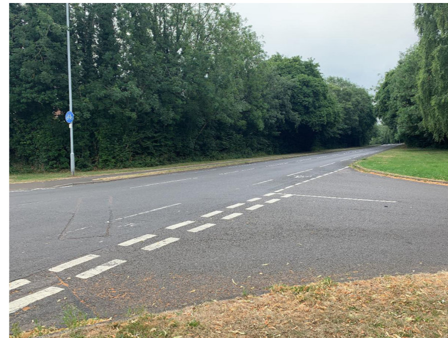
The junction radii at the junctions of Warwick Street and Staverton Road with Western Avenue encourage high traffic speeds and create hostile conditions for cycling in the carriageway.
