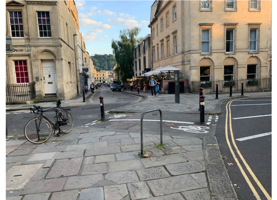
Modal filters can be used to close off arms of junctions to vehicles whilst maintaining access for people walking, wheeling or cycling
