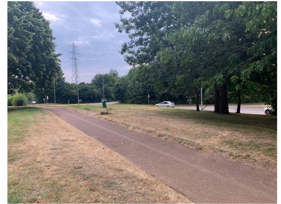
The existing cycle track adjacent to Eastern Way is in good condition but is narrow for shared use. A lack of signage means it is unclear whether the route is intended to be shared use or not.
