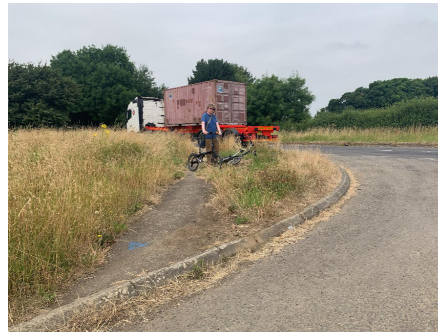
There is no crossing point on the A425 or dropped kerb on the desire line for pedestrians and cyclists.
