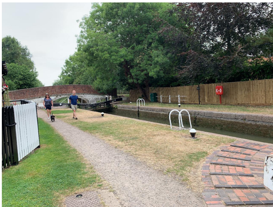
There is slightly more space at Top Lock but consideration needs to be given to accommodating boaters working the lock, walkers and cyclists here.
