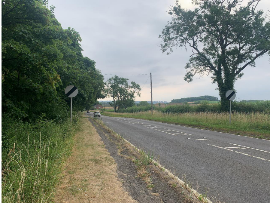
The speed limit on the A425 varies between 50mph and the National Speed Limit. There is no verge between the footway and the carriageway and the footway is in very poor condition in places.
