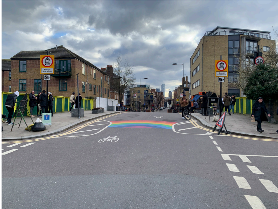
Bus gates create quiet routes for cycling in the carriageway while maintaining access for buses.
