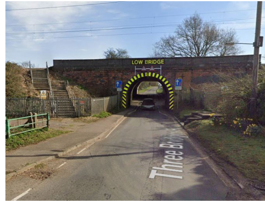
The railway bridge creates a pinch point which narrows the road down to one lane through the bridge.
