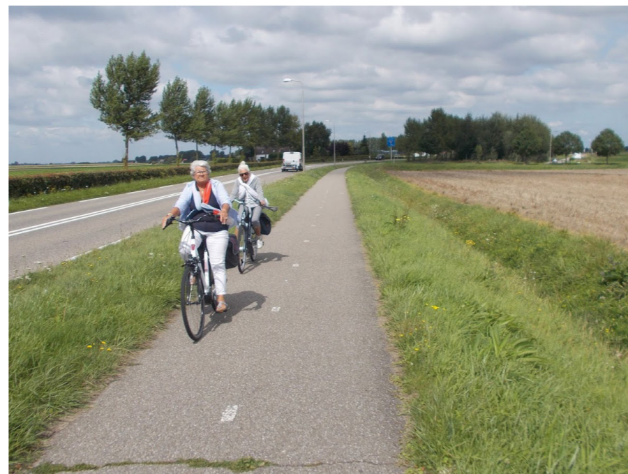
Cycle tracks that are designed for low flows of pedestrians and horse riders to share can provide a good level of service for all users on rural roads which have few or no active frontages or driveways. A buffer should be provided between the road and the shared use facility on roads with speeds over 30mph.
