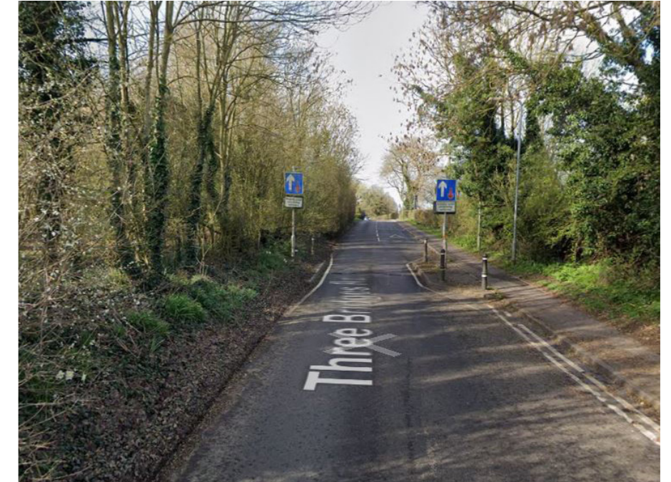
The existing pinch point west of Long Buckby Wharf acts as an effective gateway feature to slow traffic on the approach to the village.
