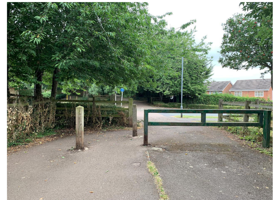
The majority of the route is accessible with very few barriers but there are a small number of bollards and barriers that need to be removed or re-sited to make the route fully accessible and reduce the risk of collisions.
