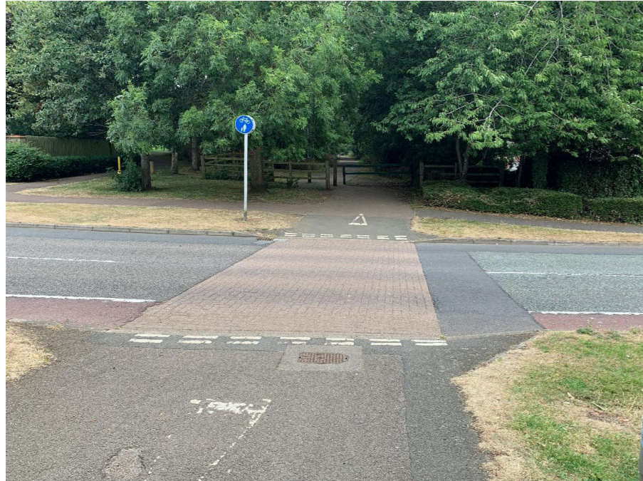
The route along the disused railway is largely grade separated from roads but crosses Shackleton Road at grade. Design priority is given to pedestrians and cyclists through the use of block paving but this is compromised by give ways on the shared use path which could cause confusion about who has priority.
