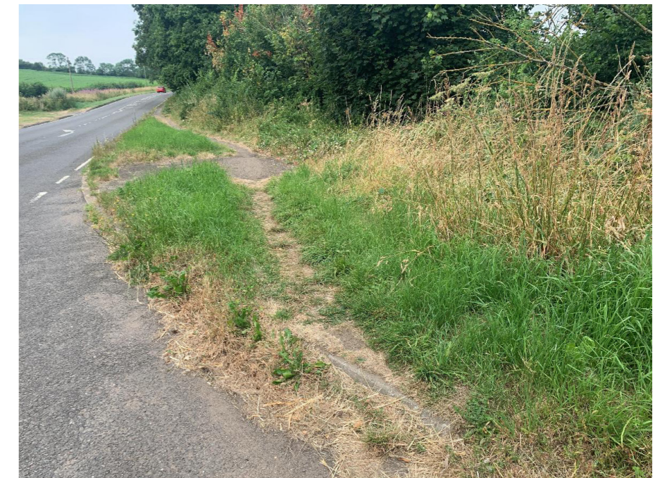
There is a significant divergence between the footway (with dropped kerb) and the desire line on the old section of Staverton Road adjacent to the A425.
