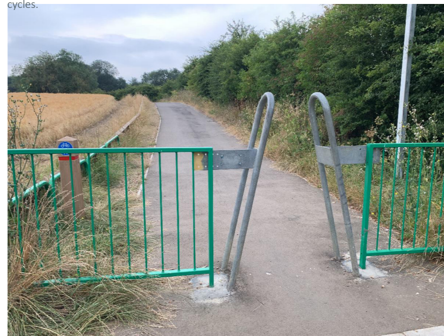
The A frame at the end of the new link means people with prams, mobility scooters and non standard cycles may be excluded from going beyond this point, including to the existing bridleway over the canal tunnel.
