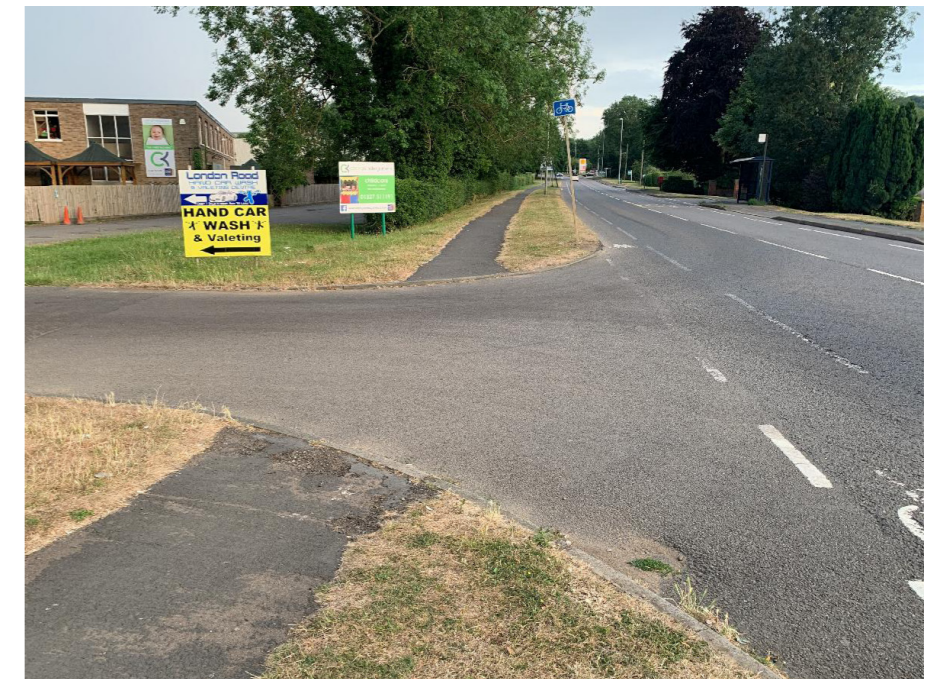
Wide radii at priority junctions along the route encourage high turning speeds, making it hazardous for pedestrians crossing side roads and for cyclists in the road.
