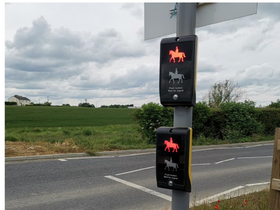
Where there is the potential for a crossing to be used by horse riders as well as pedestrians and cyclists, a Pegasus crossing should be considered to cater for all users.
