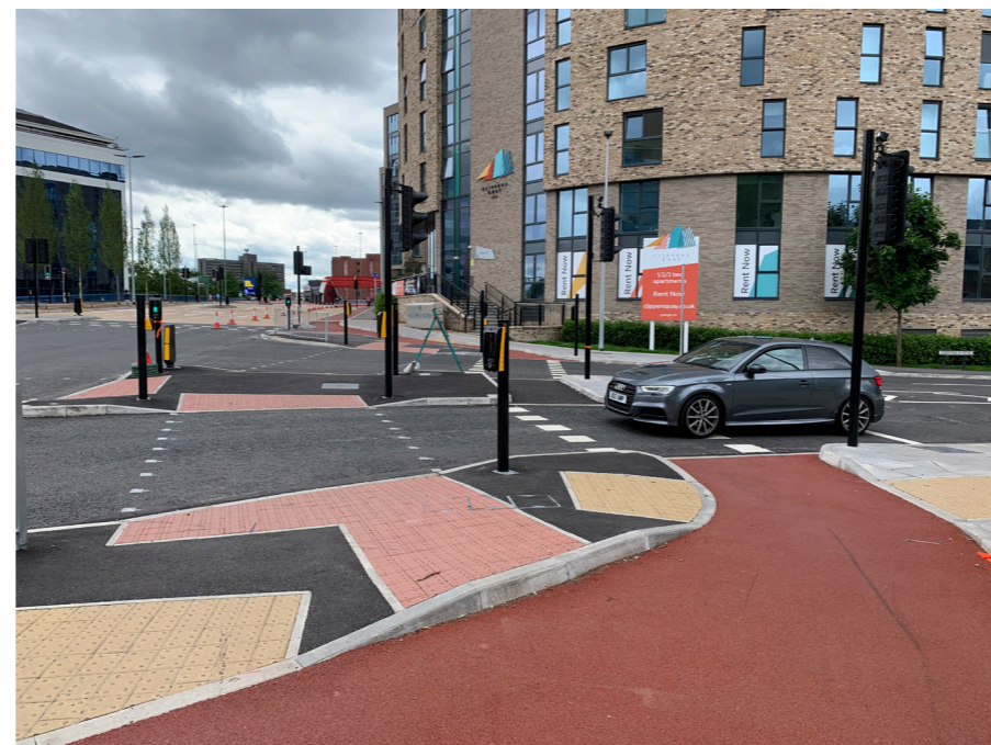
On cycle routes, it is normally best to separate pedestrians and cyclists at crossings through the provision of a parallel zebra or separate cycle signals, to reduce conflict. Cycle crossings should normally be straight across even where the pedestrian crossing needs to be staggered
