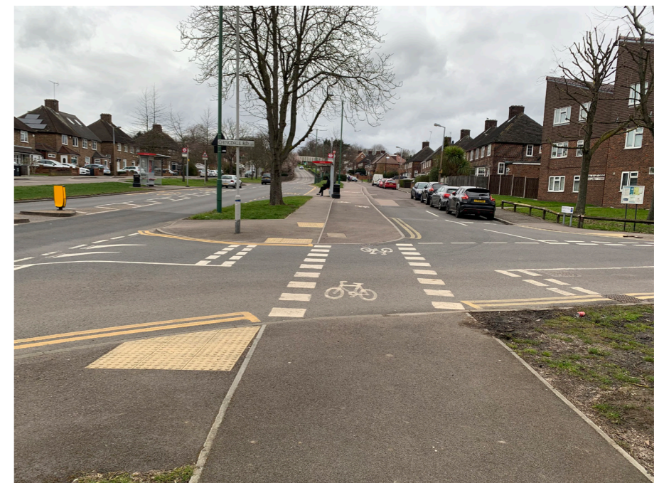
Where a two way cycle track crosses a side road, it should normally have a full set back (5 metres) with marked priority over motor vehicles using give way markings.
