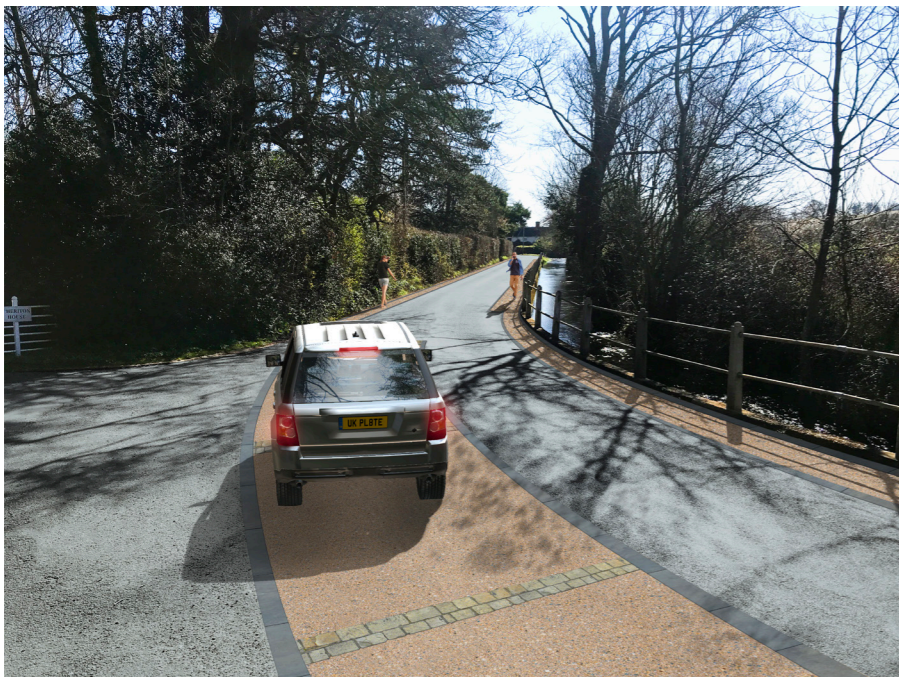
Use of different materials can mark the entrance to a place, highlighting to drivers that they need to adjust their behaviour and will have to interact with other road users
