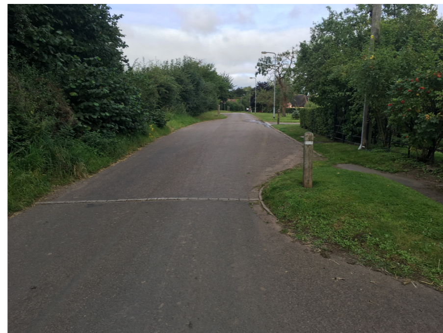
Simple pinch points can help slow traffic without detracting from the rural nature of settlements in Daventry
