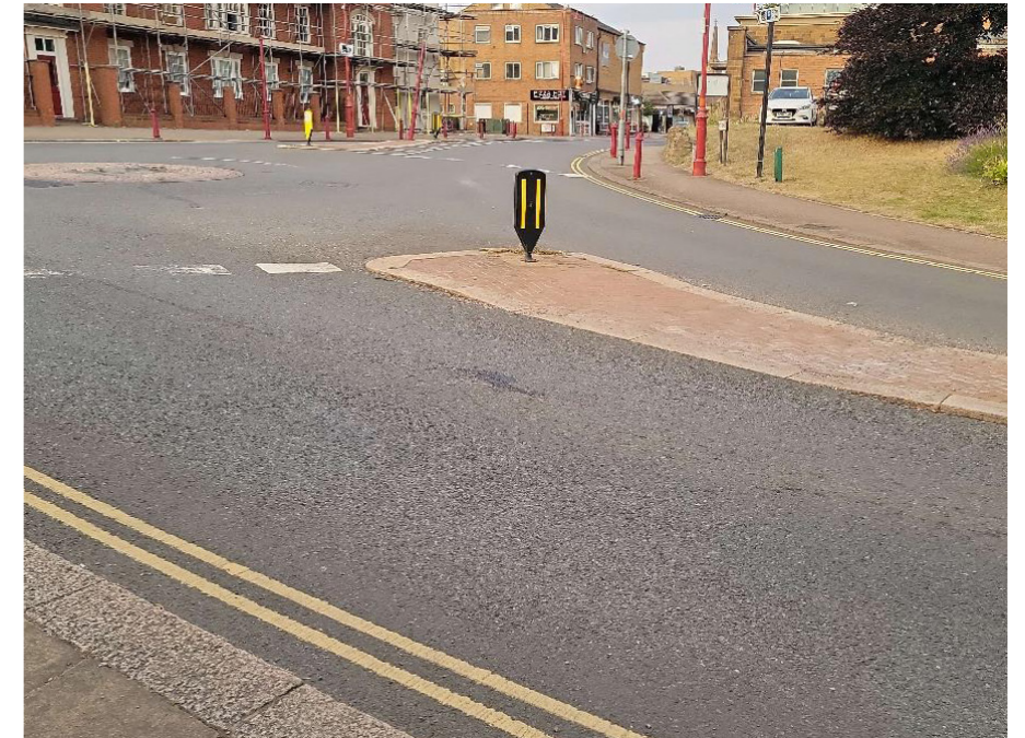
The mini roundabout at the junction of Oxford Street and London Road is awkward for cyclists to navigate and caters for higher traffic flows than is appropriate with high speeds observed in the evening.
