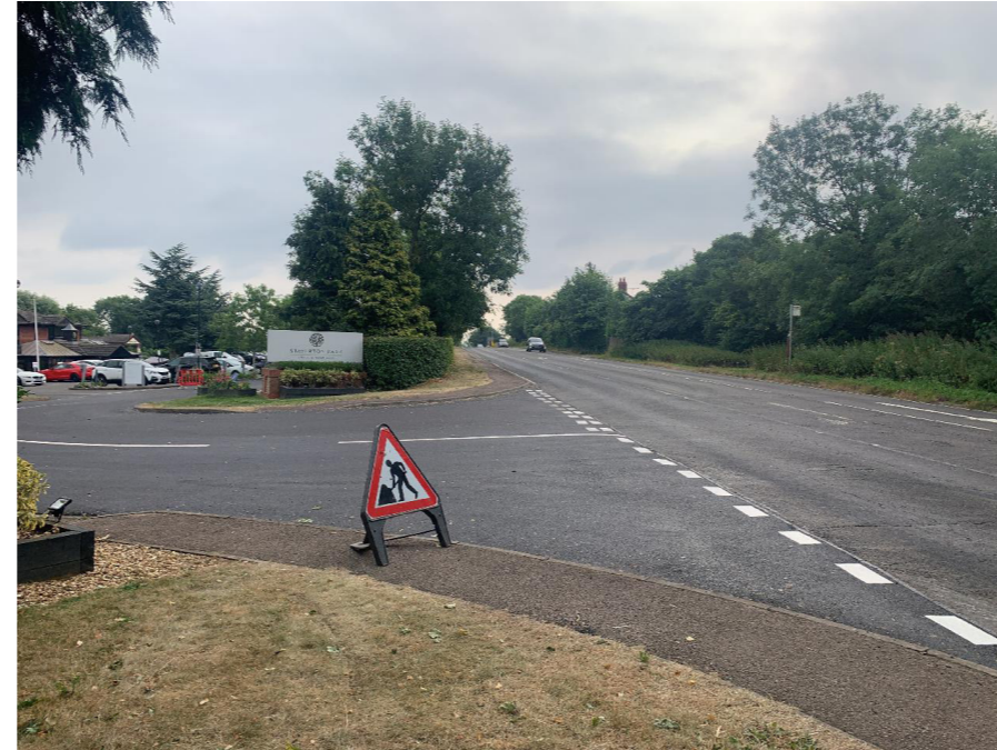
The access to the Staverton Park Hotel & Golf Club is very wide and the dropped kerbs are set well back from the desire line.
