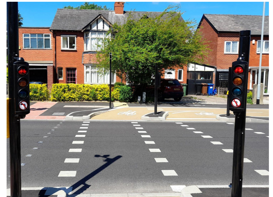
Signalised parallel crossings (Sparrow crossings) maintain separation between pedestrians and cyclists at crossing points to minimise conflict.
