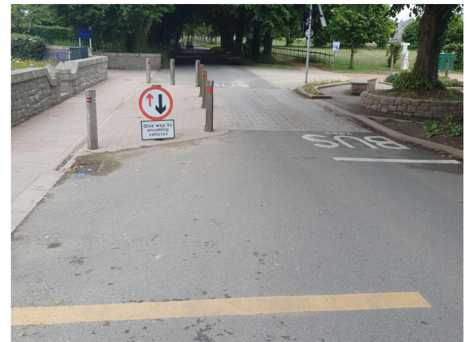
Simple pinch points can help slow traffic without detracting from the rural nature of settlements in Daventry
