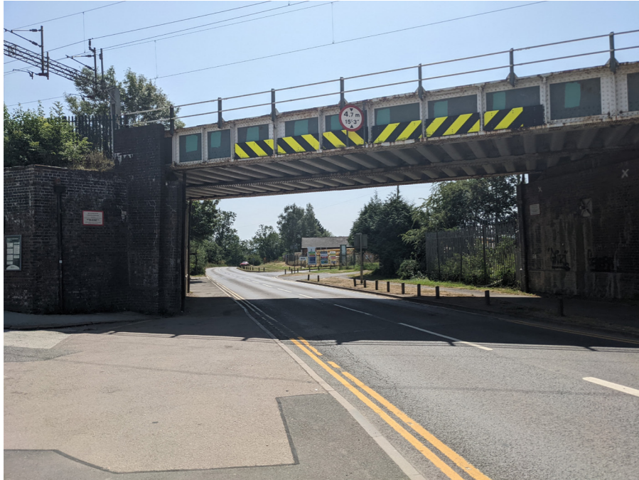
The railway bridge at Long Buckby Station creates another pinch point.
