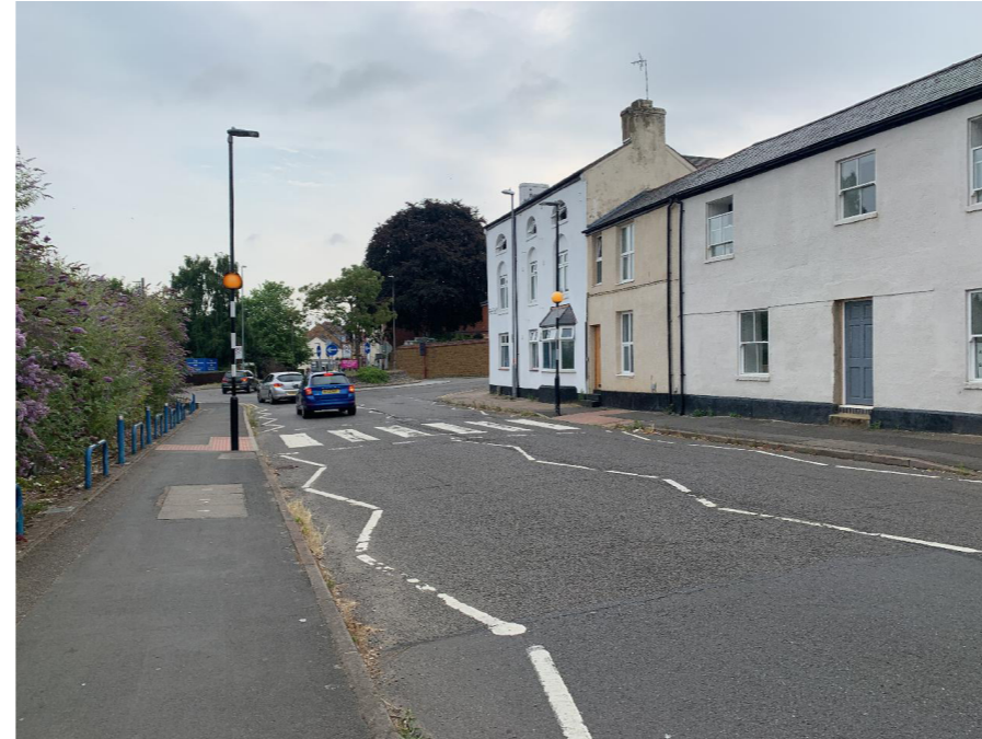
The roundabout has relatively tight geometry and zebras on two arms which help to keep speeds low
