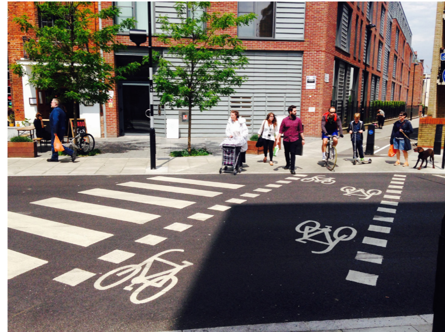
On cycle routes, it is normally best to separate pedestrians and cyclists at crossings through the provision of a parallel zebra or separate cycle signals, to reduce conflict. Cycle crossings should normally be straight across even where the pedestrian crossing needs to be staggered
