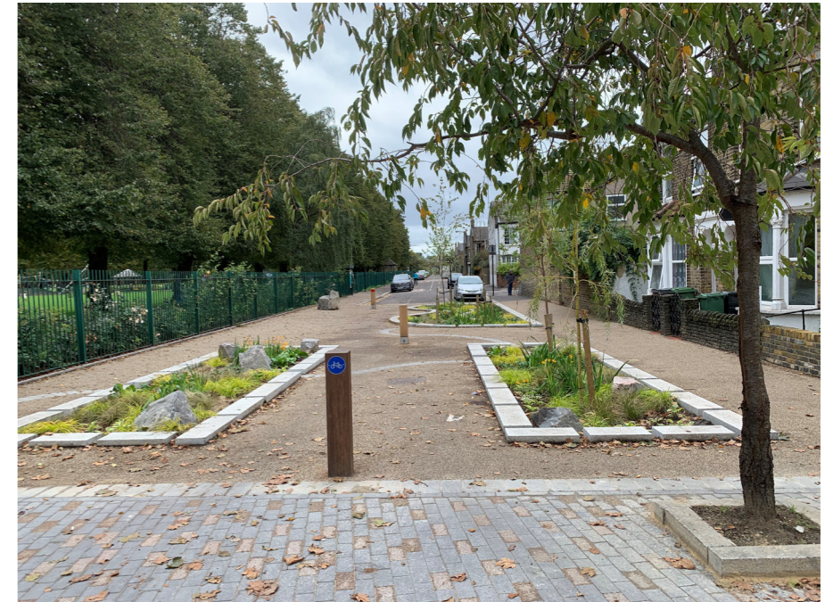
Point closures help improve conditions for walking and cycling in residential areas by reducing traffic volumes and speeds and also create space for things like street trees, rain gardens, cycle parking and even play areas.
