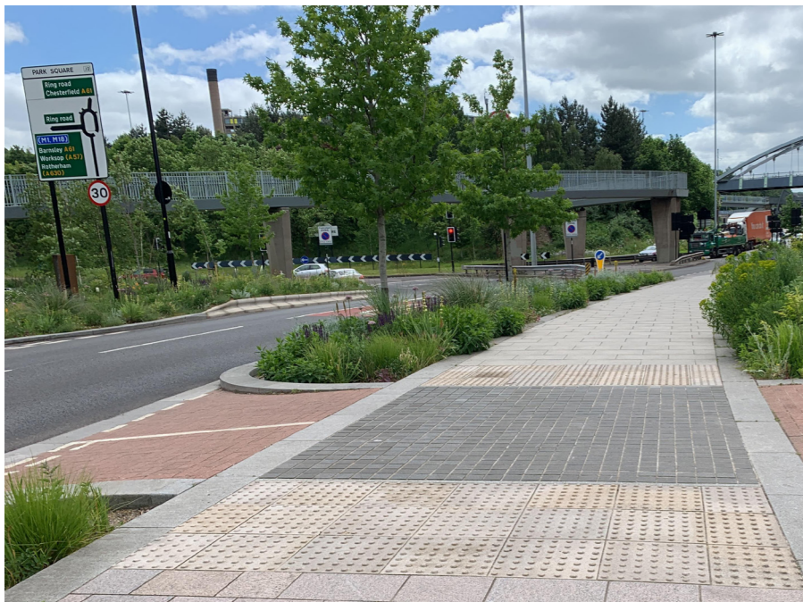
Build outs can provide a sense of arrival and space for planting while having a traffic calming affect
