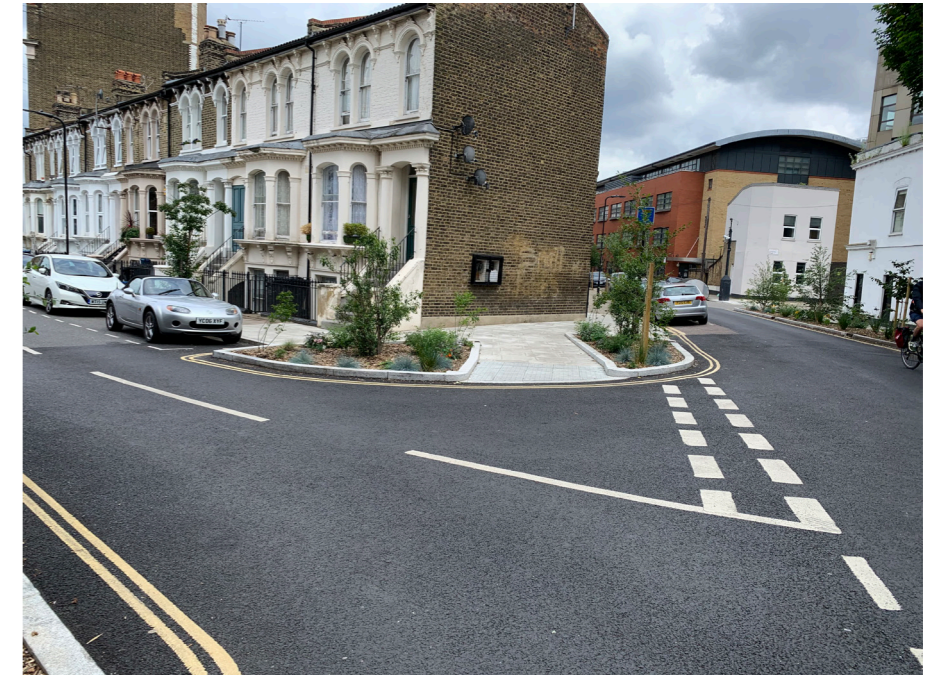
Narrowing priority junctions and overly wide carriageways can help calm traffic as well as providing space for wider footways, benches, pocket parks and formalised on-street parking.
