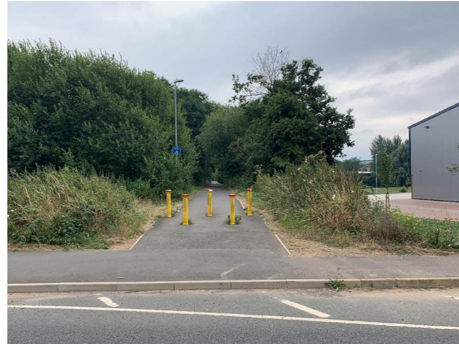
Unlike most of Daventry's traffic free network where access points are marked with two simple, slim bollards, the end of the disused railway route at Farnborough Drive has five large bollards which make the route difficult to access for people with prams or non-standard cycles.
