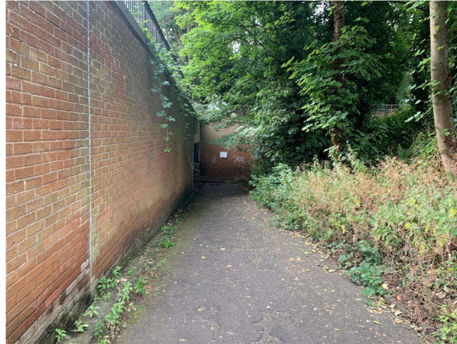
Unlike most subways in Daventry, sight lines on the other side of the subway are poor from the ramp which is likely to mean people avoid using it due to personal safety fears.
