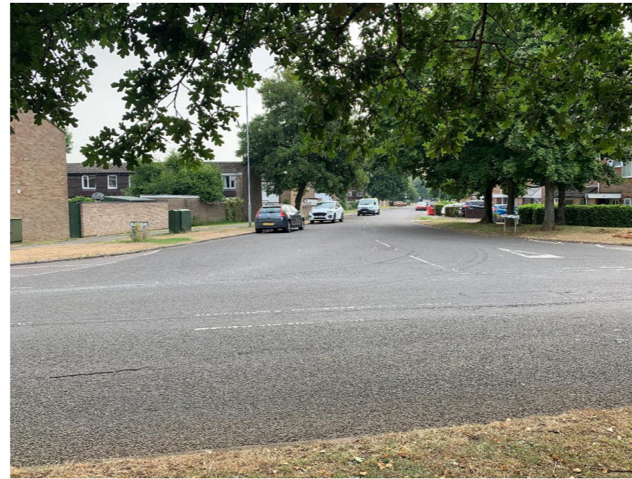
The junction of Staverton Road and Thames Road is excessively wide even with painted hatching to visually narrow the junction. This is likely to encourage higher vehicle speeds and make it difficult for people walking and cycling to cross the road to the bridge.
