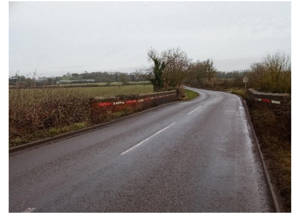
The three Surney bridges on Three Bridges Road create pinch points where there is insufficient space to provide protected space for cycling immediately adjacent to the carriageway.
