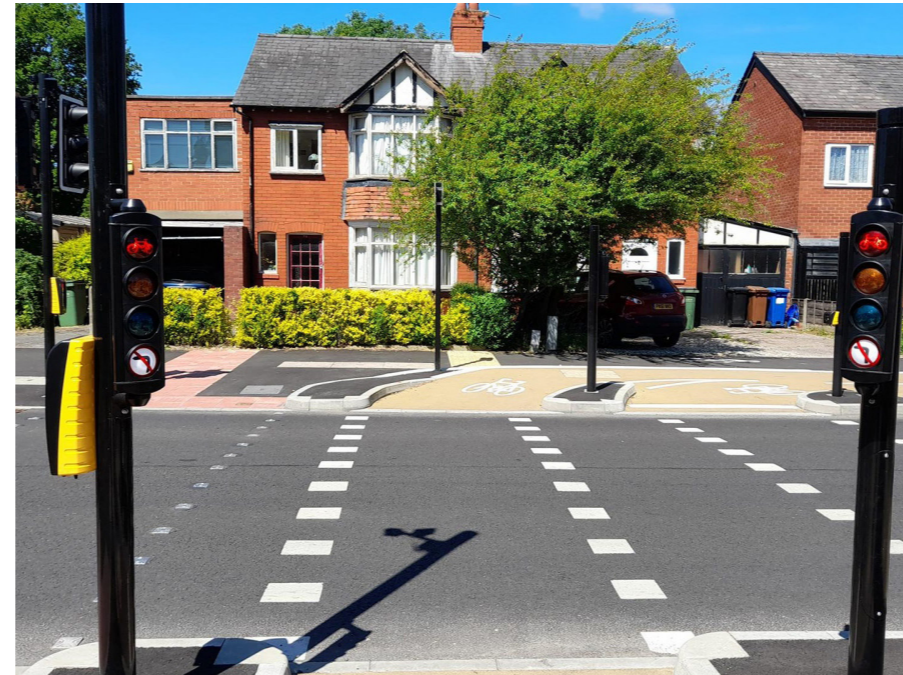
Signalised parallel crossings (Sparrow crossings) maintain separation between pedestrians and cyclists at crossing points to minimise conflict.
