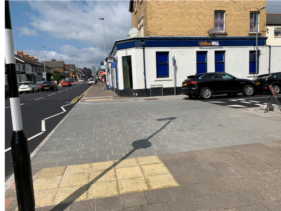
Continuous footways provide priority for pedestrians over cars in areas of high footfall (Cardiff)
