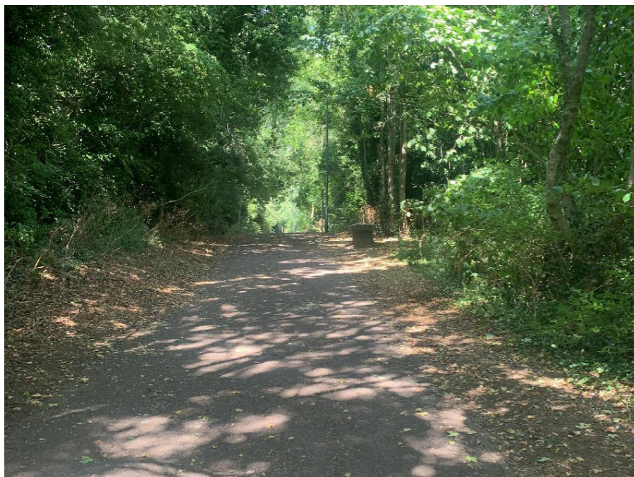
The route along the disused railway line is generally in good condition, has a bitmac surface, street lighting and good wayfinding along it.
