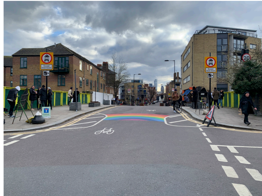
Bus gates create quiet routes for cycling in the carriageway while maintaining access for buses.
