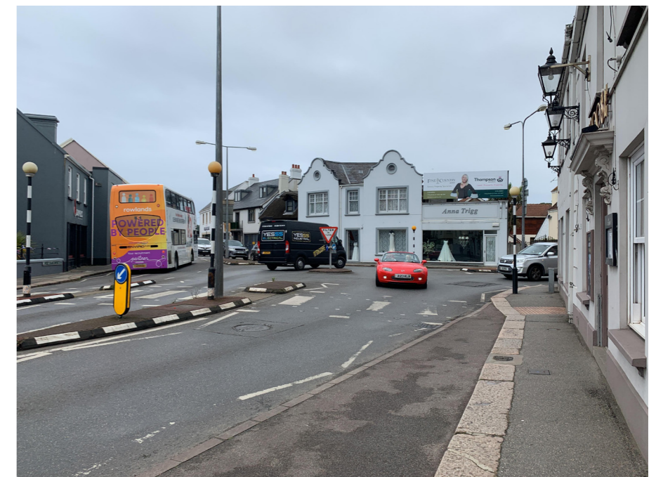
Filter in turn junctions provide a good alternative to mini roundabouts and create low speed environments suitable for providing pedestrian crossings
