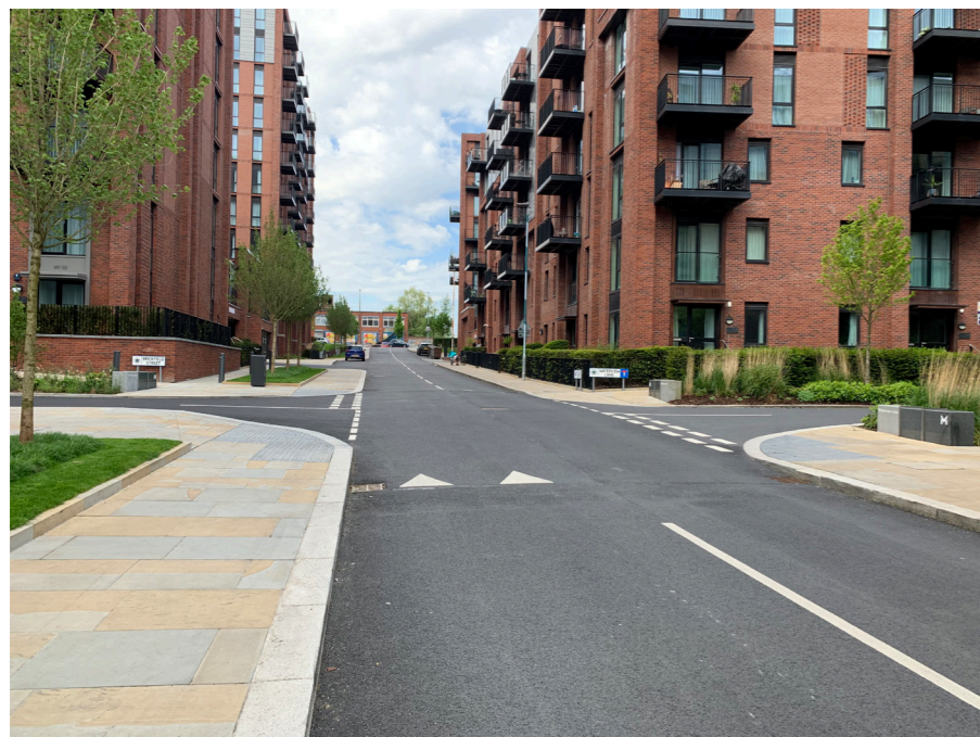
Tightening priority junctions and installing raised tables improves safety for pedestrians and cyclists by reducing crossing distances and vehicle speeds.
