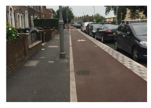
Constructing cycle tracks at (or close to) footway level can be a good solution where space is very constrained (Waltham Forest)
