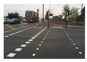
Complex <u>junction improvements</u> involve redesign of the junction geometry and provision of a signalised crossing
