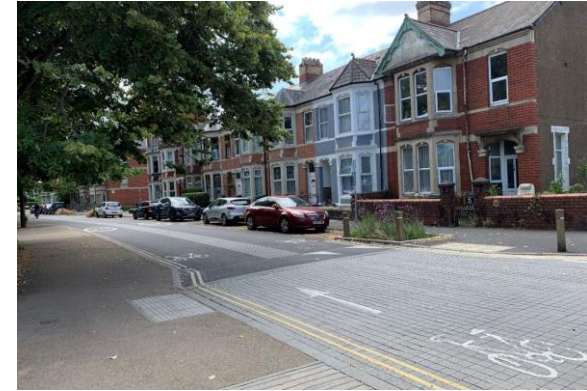
Design cues such as cycle symbols in the carriageway, raised tables and build outs can help slow traffic
