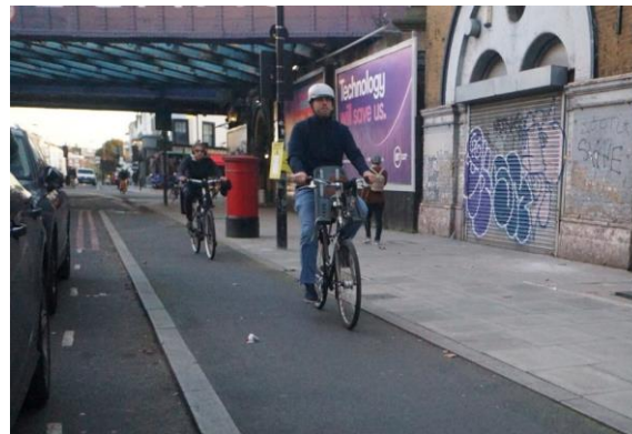
Protected cycle tracks can be 'stepped' or run behind parking to improve space efficiency.
