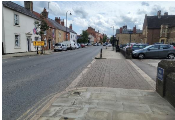
Continuous footways and tightened junction radii can slow turning traffic (example from Towcester Police Station)
