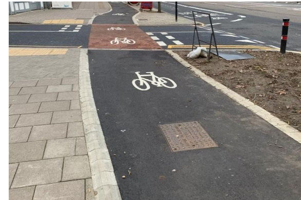
Providing priority over side roads is an easy way of improving the existing cycle network – also helps pedestrians
