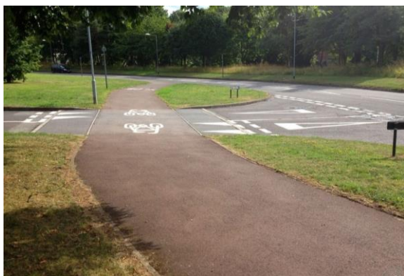
Set-back cycle priority at side roads can provide a smoother journey for cyclists (and pedestrians)
