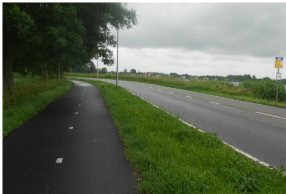
Bi-directional cycle tracks which pedestrians and horse riders can also use are commonplace in Europe in low footfall areas.
