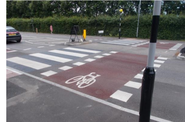
Parallel crossings give priority to both pedestrians and cyclists in lower traffic/speed areas.
