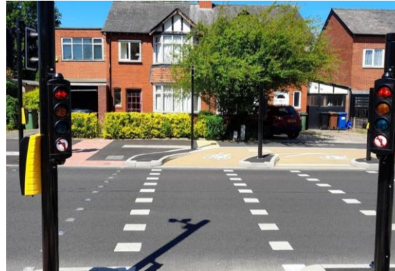
Signalised parallel crossings (Sparrow crossings) maintain separation between pedestrians and cyclists at crossing points to minimise conflict.
